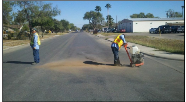
Crews working at Yoakum Street
