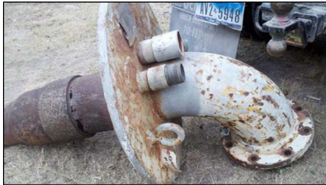
Old Well head with 8" pipe at well #14
