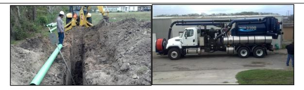
Wastewater Crews are installing 400 feet of Sanitary Sewer line at 900 Block of Dodridge.
