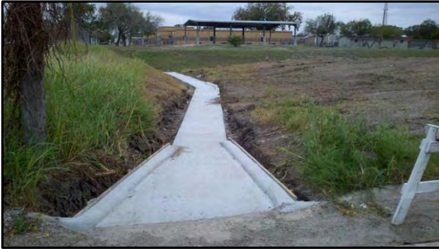
New Concrete flume at Ave B
