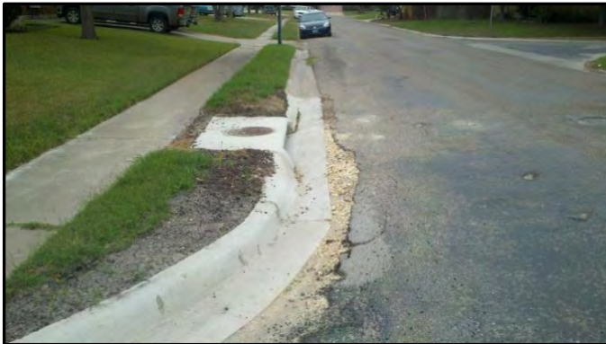
New Curb & gutter and Inlet at 21th and Warren
