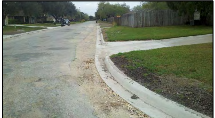
New Curb & gutter and Inlet at 21th and Warren
