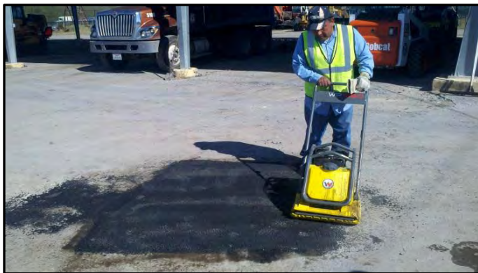
Compaction after the filling up the pothole
