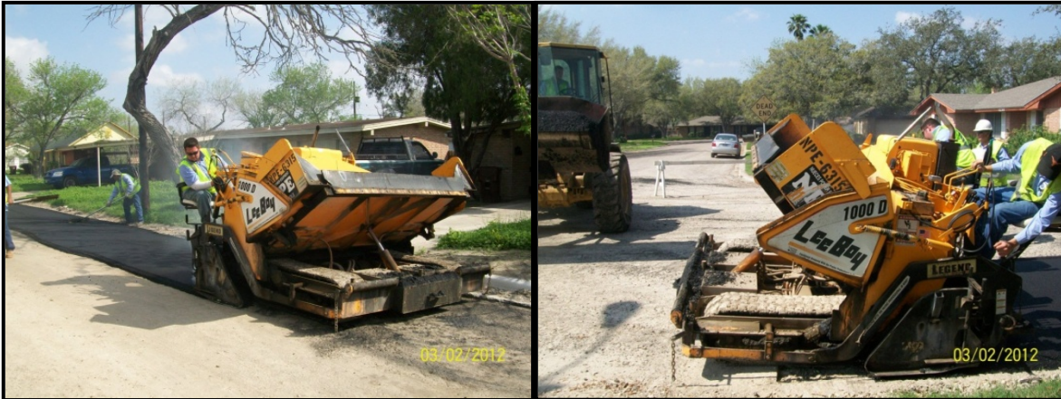
Street Division Crews are working at Lawndale area.
