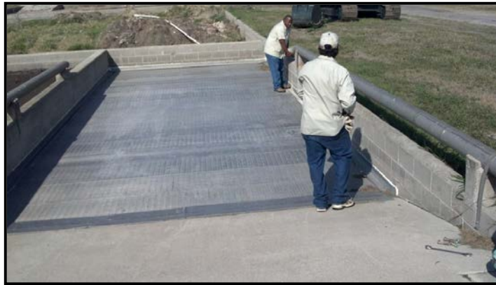
Wastewater crews are working on Sludge Discharge pipe at North Treatment Plant
