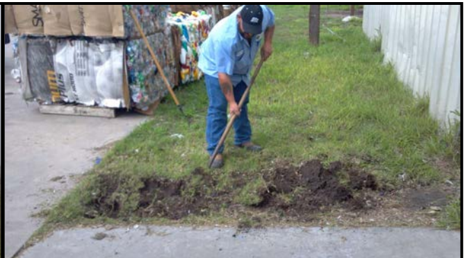
Sanitation crew is doing dirt work to construct a concrete pad for the Compactor at Recycling Center.
