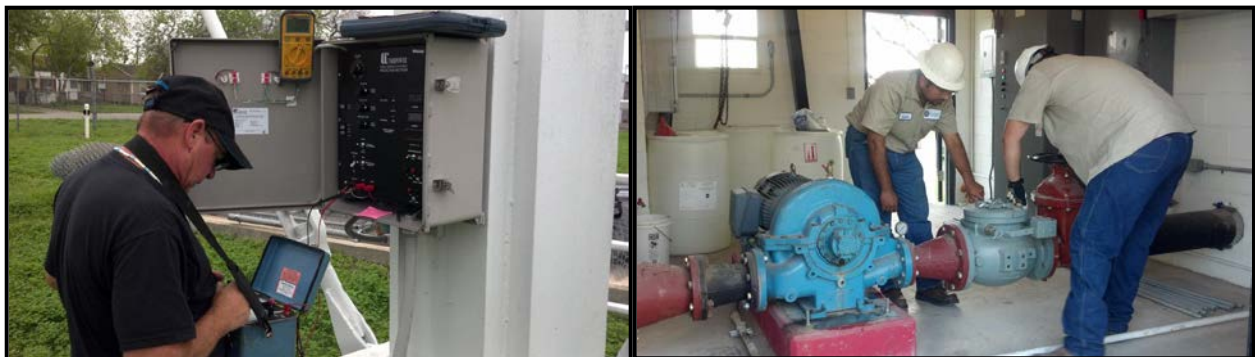
Contractor is performing annual inspection of Cathodic Protection systems on Tanks Water Production crews are doing maintenance on 8" check valve at well no. 23
