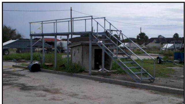
Catwalk for Car Wash
