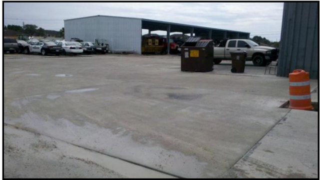
New Pavement in front of the City Garage
