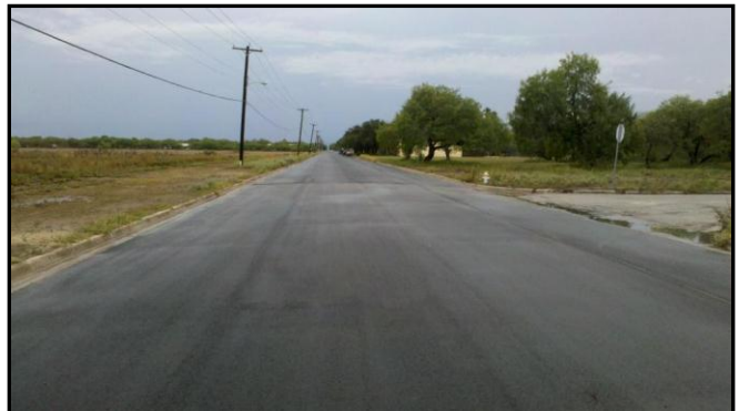
HMAC pavement reconstruction is done
