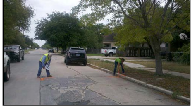
Staff marking the areas to be repaired
