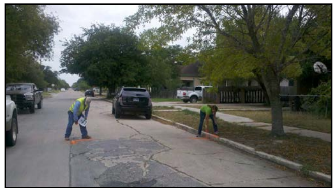
Staff is marking the areas to be repaired
