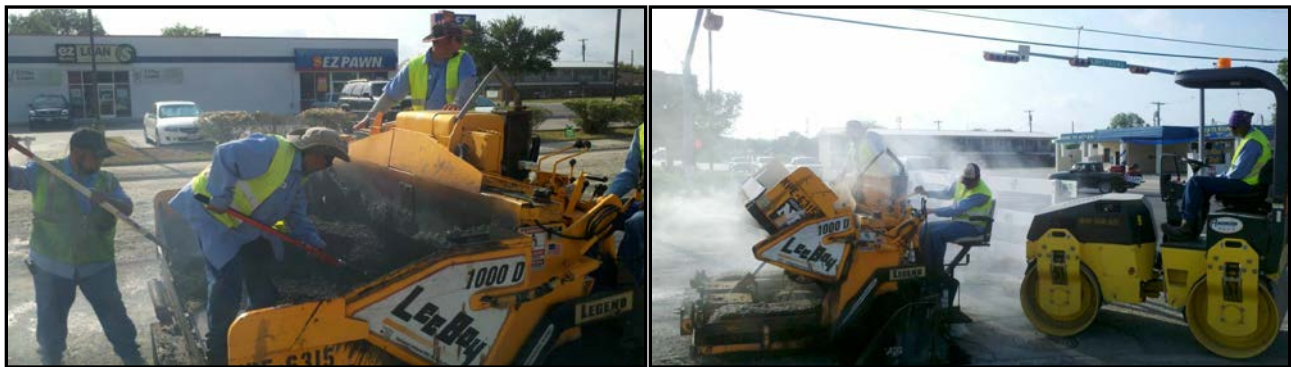
Crews are working on Armstrong Paving Project
