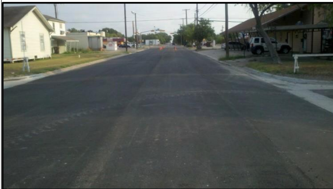
Street Division crews worked at Armstrong Ave.
