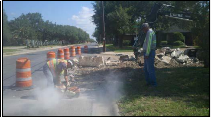
Contractor is working at Henrieta and Armstrong (from Huisache to Johnston) Intersection
