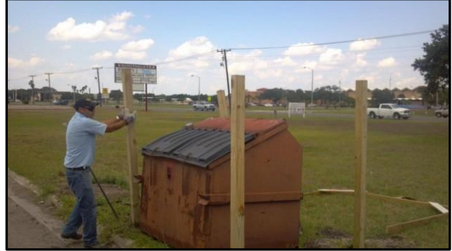
Installation of dumpster enclosure by the contractor. The City's Sanitation Supervisor is the project manager for the dumpster enclosure pilot program
