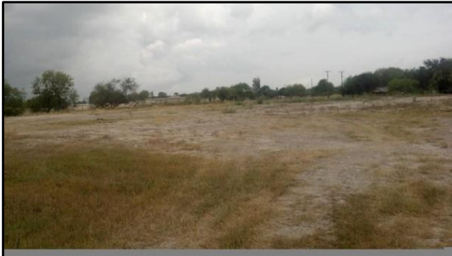
Dirt was removed from 17 th and Lee
