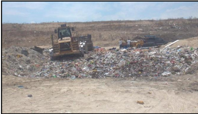
Landfill Working Phase
