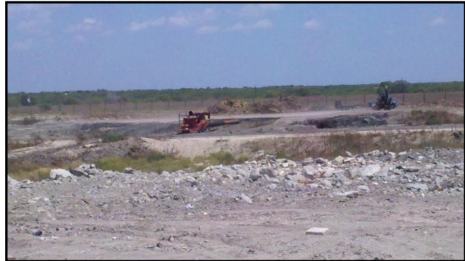
Burner is working
