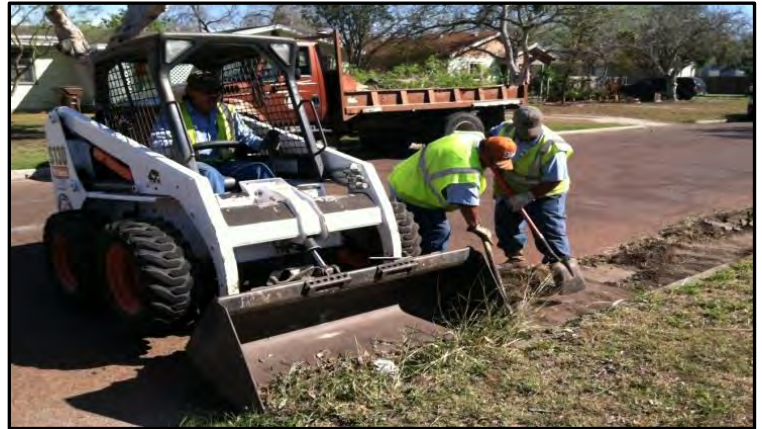
Street crews are cleaning curb & gutter Street at Shelton
