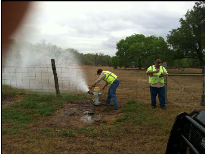
Flushing water lines for increased residual.
