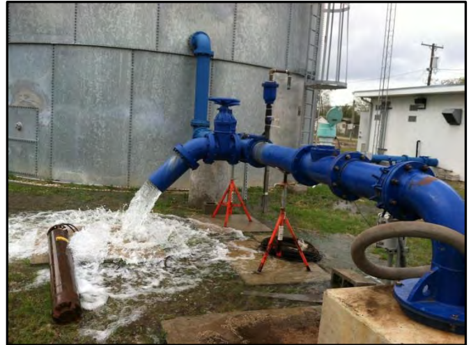
Disinfecting Well #24 after pump repairs
