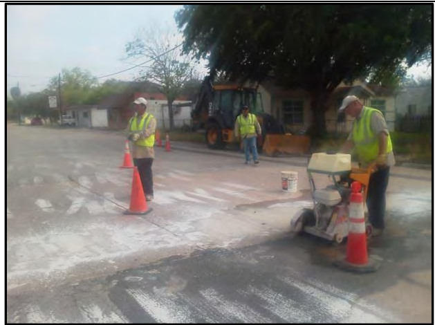
Preparing concrete for new waterline crossing
