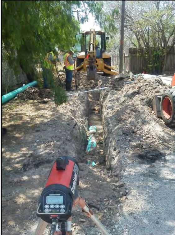
Wastewater crew replacing failing sewer line at Armstrong and Yoakum
