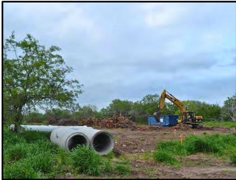
New Drainage on Campus
