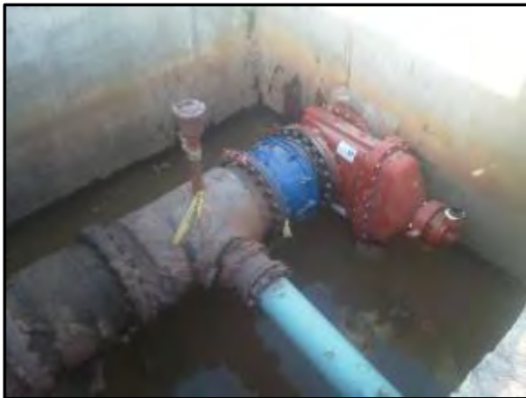
18" valve replacement, 2 of 4 complete
