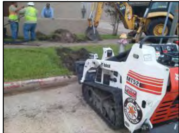
Utilizing new trenchless boring attachment
