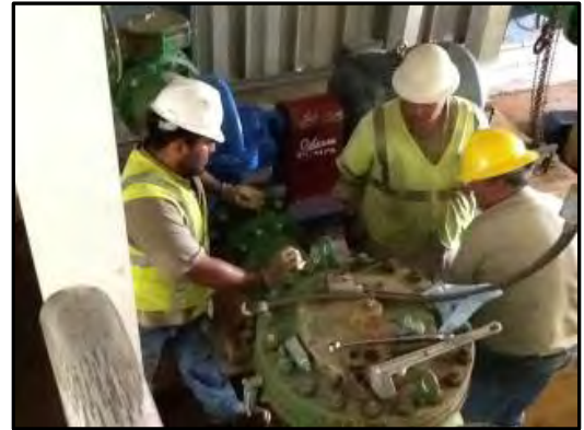
Removing power actuated control valve at STWA
