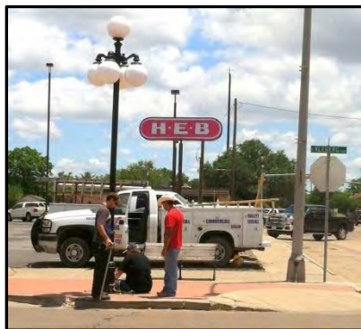
Replacing Street Lamp
