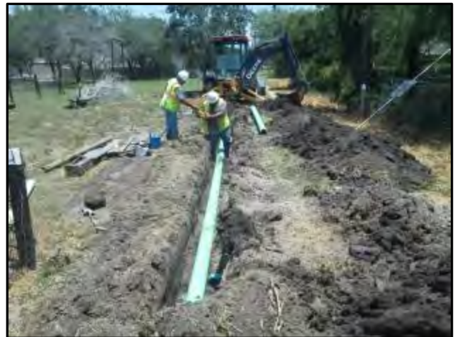
Replacing 500 lf of sewer main at 900blk of W. Yoakum
