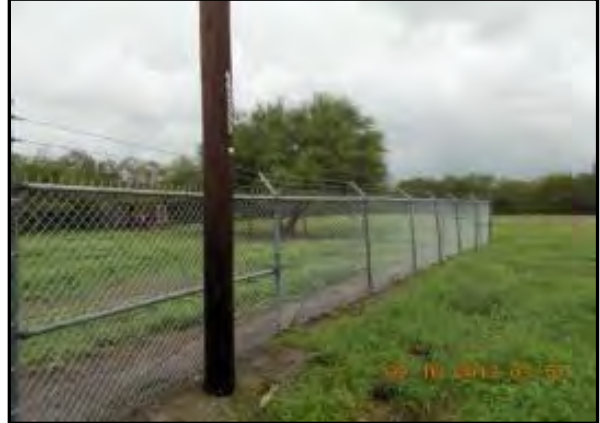
New fence line with 3 strand barbed wire
