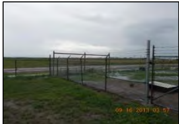
New fence line with 3 strand barbed wire
