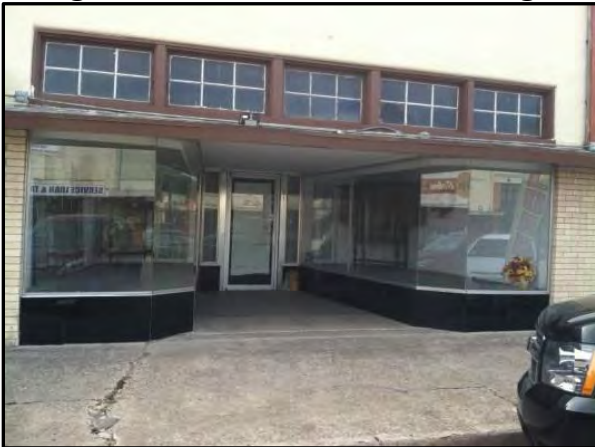
New glass installed at 313 East Kleberg
