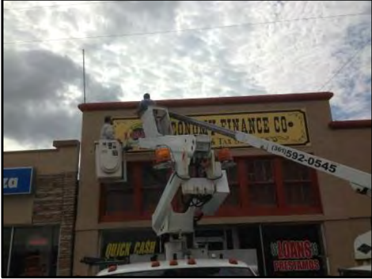
New Sign for Economy Finance was installed
