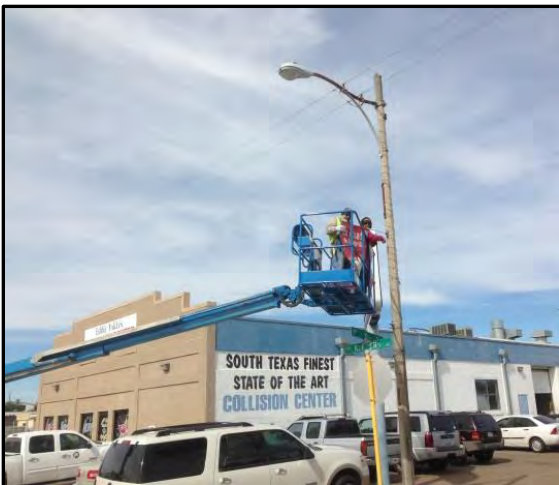
La Posada Banners and Christmas decorations are being installed
