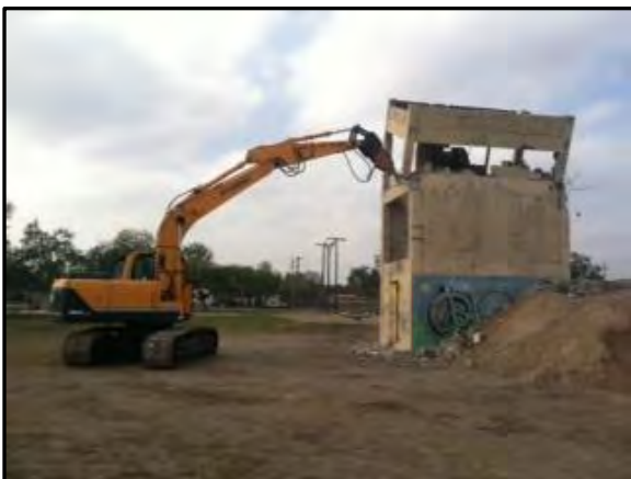
Garage department removes steel on the structure (street department assist) Garage department welds metal plates to attach the hydraulic hammer
