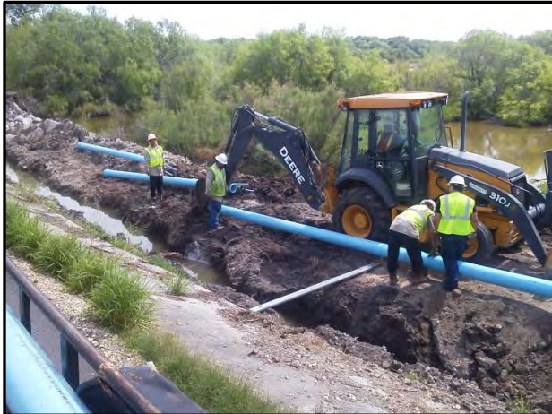
CR 1030 waterline extension
