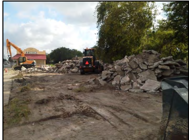
Apple House slab demolition
