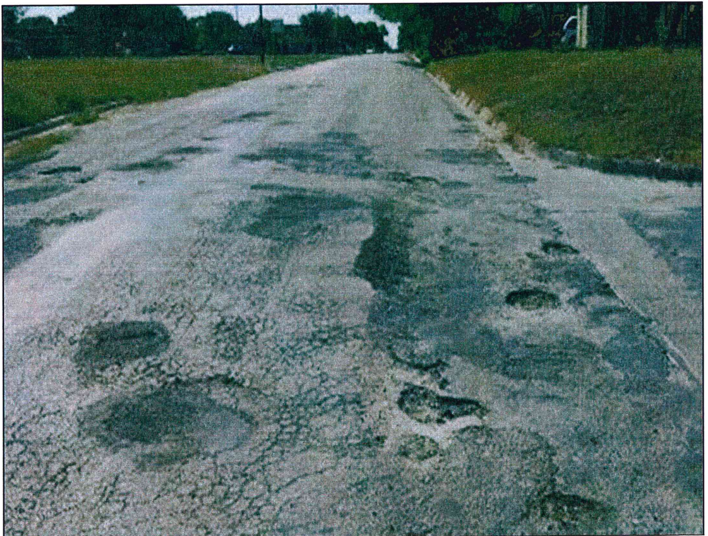
Poor- Asphalt (12 th Street)
