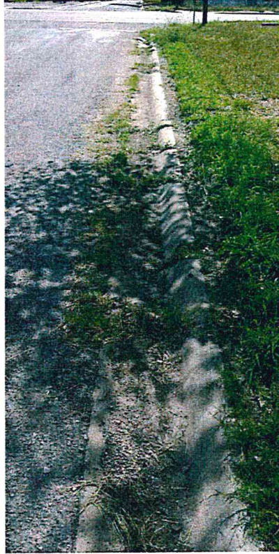
Poor - Rollover Curb
