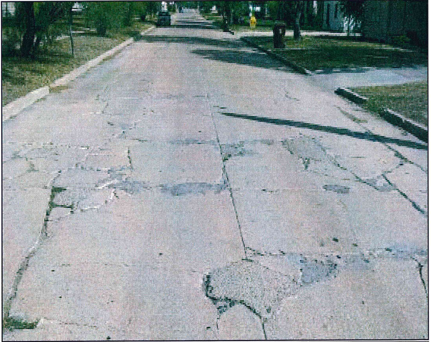
Poor - Concrete Street
