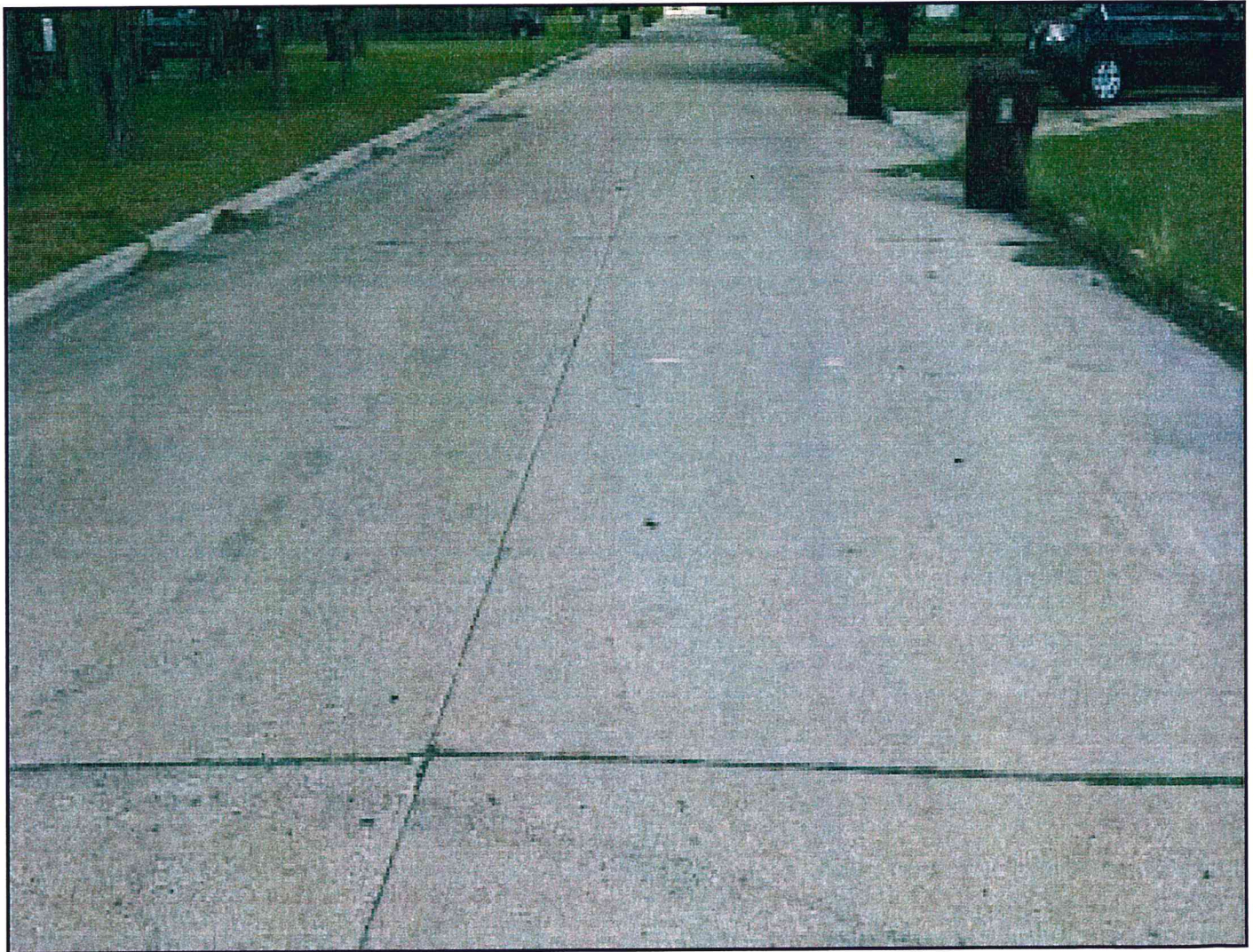
Good- Concrete Street
