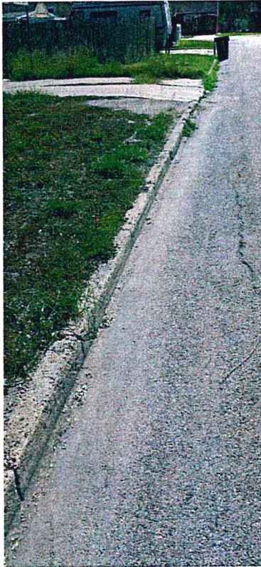
Poor – Square Curb
