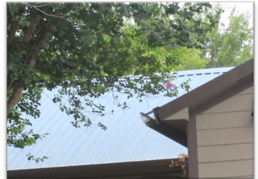
“V” CRIMP ROOFING
