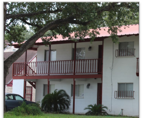
TWO-TIERED FRONT PORCH WITH FIRST FLOOR AT GROUND LEVEL
