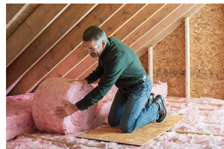
FIBERGLASS BATT IS AN APPROPRIATE INSULATION MATERIAL
