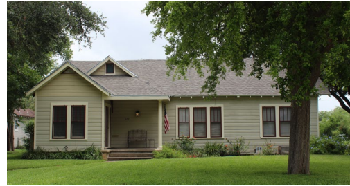
FRONT FACING GABLE ON CROSS GABLE ROOF WITH BOXED EAVES
