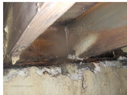
SPRAY INSULATION IS NOT RECOMMENDED SINCE IT CAN TRAP MOISTURE AND MASK WATER LEAKS, CAUSING WOOD TO ROT
