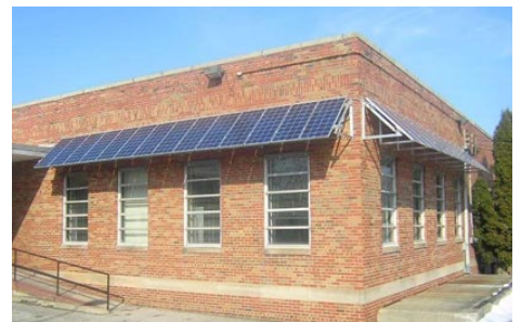
SOLAR PANELS, WHICH ALSO SERVE AS AWNINGS, WERE INSTALLED IN SECONDARY LOCATIONS ON THE SIDE AND REAR OF THIS HISTORIC POST OFFICE AND CANNOT BE SEEN FROM THE FRONT OF THE BUILDING. (SOURCE: NPS)
