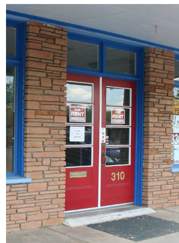
CUT STONE ON FAÇADE OF BUILDING
