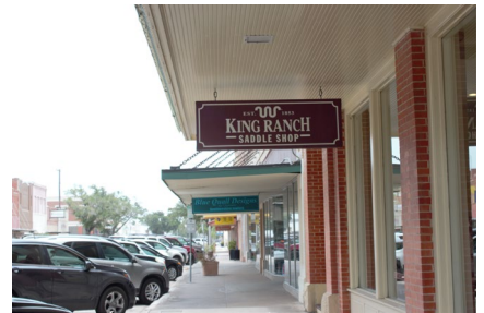
CANOPIES PROTECTING PEDESTRIAN WALKWAYS
