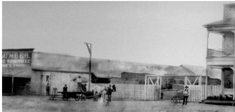
KINGSVILLE'S LUMBER AND HARDWARE STORE BEFORE 1909.
