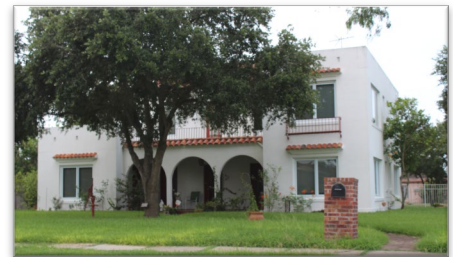
STUCCO AS EXTERIOR WALL SURFACE
