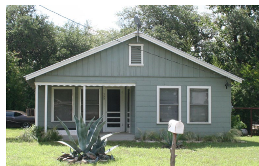
ASBESTOS SHINGLES DO NOT TRAP MOISTURE BUT CAN ALTER THE HISTORIC APPEARANCE OF A HOUSE
