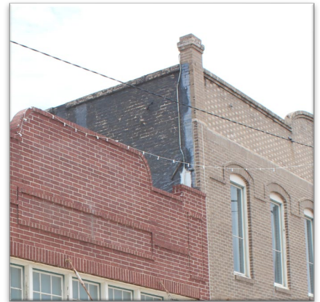
SIDE FAÇADE MATERIALS OFTEN DIFFER FROM THE FRONT FACADE
