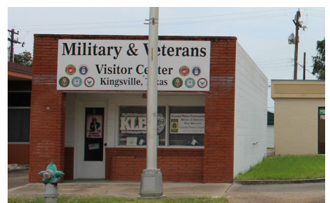
COMMERCIAL BUILDING WITH BRICK FRONT AND CMU SIDES
