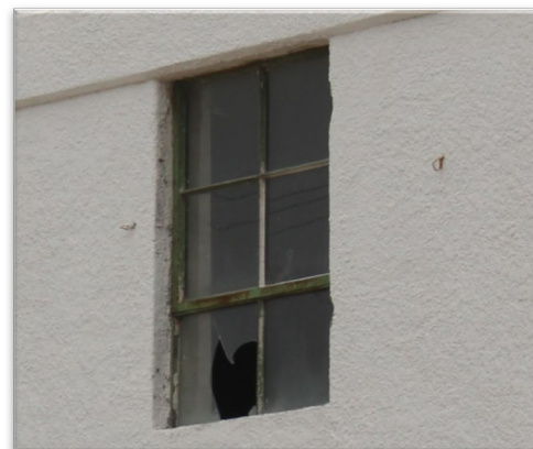
BROKEN GLASS SHOULD BE REPLACED IMMEDIATELY TO AVOID FURTHER DAMAGE
