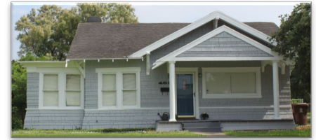
A HOUSE WITH WOOD SHINGLE SIDING
