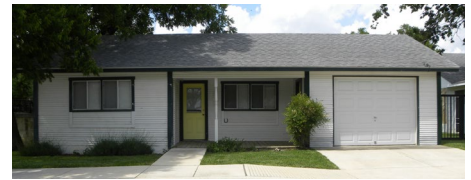
COMPOSITION SHINGLE ROOFING
