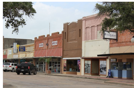
BUILDINGS FOLLOW A COMMON LINE OF CONSTRUCTION
