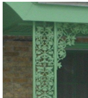
FABRICATED METAL COLUMN
