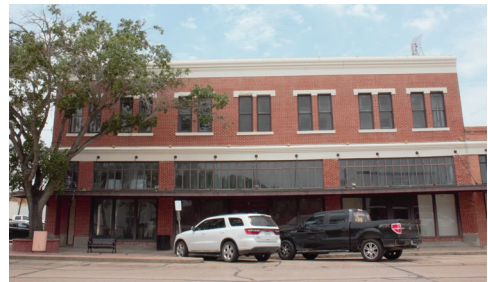
PUNCHED OPENINGS ARE COMMON AT UPPER FLOORS
