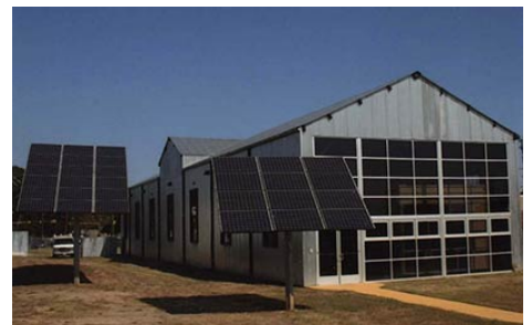
FREE-STANDING SOLAR PANELS HAVE BEEN INSTALLED WHERE THEY ARE VISIBLE BUT APPROPRIATELY LOCATED AT THE REAR OF THE PROPERTY AND COMPATIBLE WITH THE CHARACTER OF THE BUILDING. (SOURCE: NPS)
