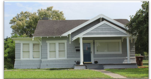
WOOD SHINGLE SIDING AND SKIRTING
