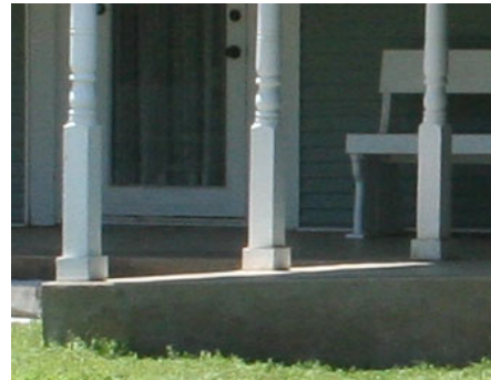
BASE OF A COLUMN
