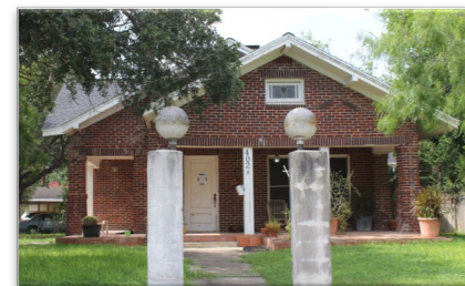
IT IS IMPORTANT TO RETAIN AND MAINTAIN BRICK. IF MORTAR SHOULD BE REPLACED IT SHOULD MATCH IN COMPOSITION, COLOR, AND JOINT WIDTH
