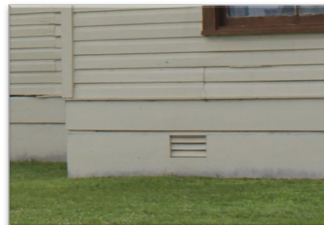
SKIRTING SHOULD HAVE VENTILATION TO PREVENT TRAPPING MOISTURE
