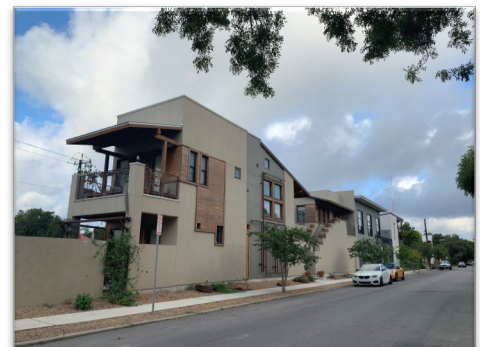
NEW CONSTRUCTION HAS SIMILAR SCALE, RHYTHM AND PROPORTIONS TO BUILDINGS AROUND IT.
