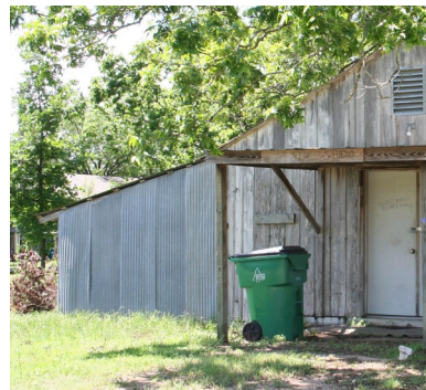
SHED ROOF ON OUTBUILDING
