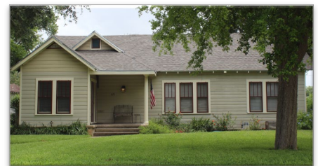
HORIZONTAL WOOD SIDING ON A HOUSE WITH CORNER BOARDS AND WINDOW TRIM INTACT.
