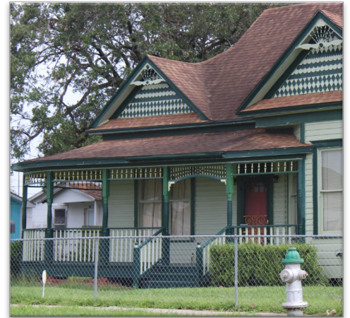
PORCHES ARE A PROMINENT FEATURE OF A HOUSE AND SHOULD BE PRESERVED
