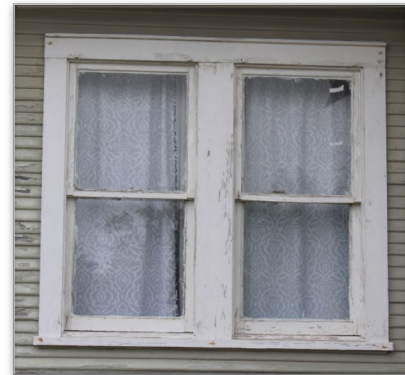
DOUBLE HUNG WOODEN WINDOWS PLAY AN IMPORTANT ROLE IN THE CHARACTER OF THE HOUSE
