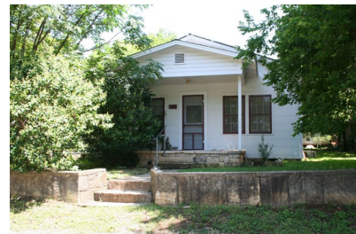
RETAINING WALL IN FRONT OF A HOUSE
