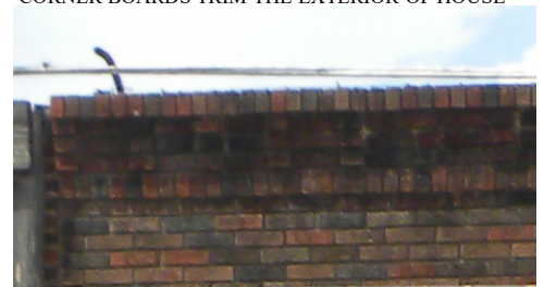
BRICK CORNICE AT TOP OF WALL
