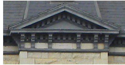
DENTILS ON CORNICE AND EAVE
