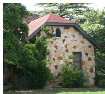
CLIPPED GABLE ON FAÇADE OF HOUSE
