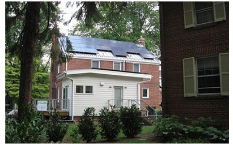
NOT RECOMMENDED - SOLAR ROOF PANELS HAVE BEEN INSTALLED AT THE REAR, BUT BECAUSE THE HOUSE IS SITUATED ON A CORNER, THEY ARE HIGHLY VISIBLE AND NEGATIVELY IMPACT THE CHARACTER OF THE HISTORIC PROPERTY. (SOURCE: NPS)
