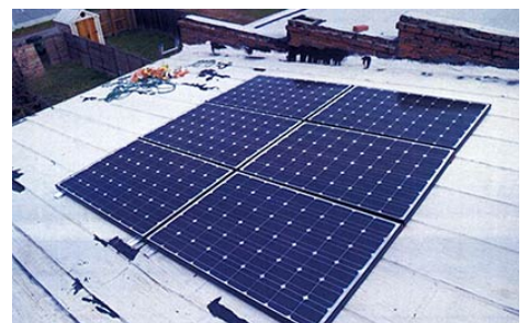
SOLAR PANELS WERE INSTALLED APPROPRIATELY ON THE REAR PORTION OF THE ROOF ON THIS HISTORIC HOUSE THAT ARE NOT VISIBLE FROM THE PRIMARY ELEVATION. (SOURCE: NPS)
