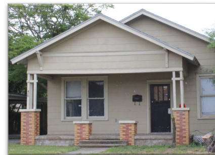
IT IS IMPORTANT TO PRESERVE BRICK DETAILING BECAUSE IT ADDS TO THE CHARACTER
