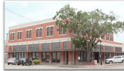
COMMERCIAL BRICK BUILDING
