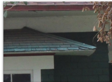
WOOD SHINGLES ON A RESIDENTIAL CANOPY
