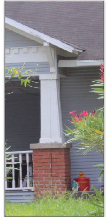
BRICK IS VERY COMMON AS A BASE TO TAPERED COLUMNS
