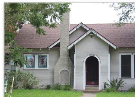
HOUSE WITH HORIZONTAL WOOD SIDING
