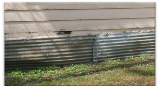
METAL SKIRTING SHOULD NOT BE INSTALLED WERE IT DID NOT PREVIOUSLY EXIST
