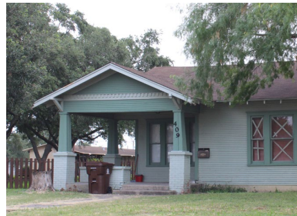
PORCH WITH TAPERED BOX COLUMN SUPPORTS
