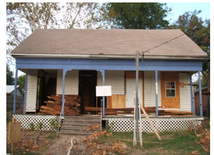
WHEN REPLACING DOORS AND WINDOWS, MATCH ORIGINAL, DO NOT CHANGE STYLES.
