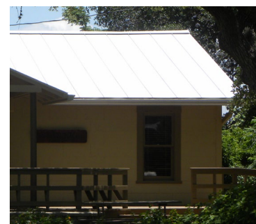
STANDING SEAM METAL ROOFING
