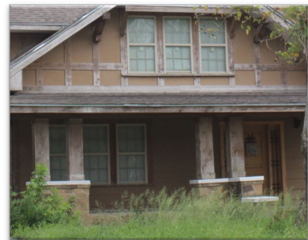
STONE ON COLUMN PIERS
