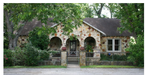
HOUSE MADE FROM STONE RUBBLE
