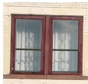
MULLION BETWEEN THE WINDOWS
