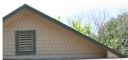
WOOD SHINGLES ON A HOUSE
