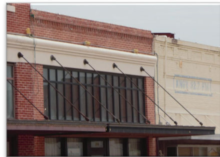
METAL CANOPY TIE-BACKS
