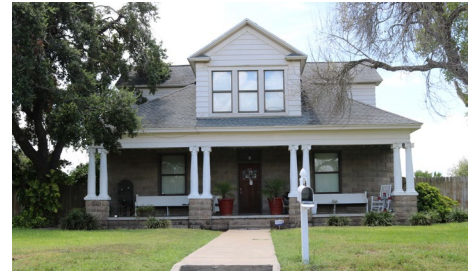
HOUSE WITH UNPAINTED RUSTICATED FACE BLOCK
