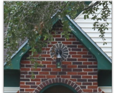
ORIGINAL LIGHT FIXTURE ABOVE FRONT DOOR
