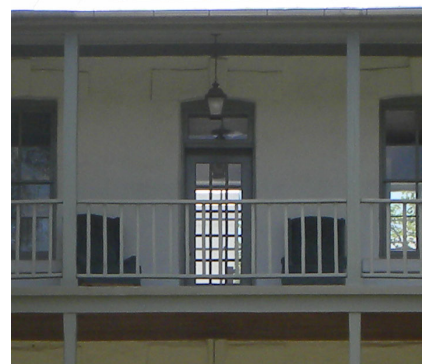
BALUSTRADE ALONG EDGE OF PORCH
