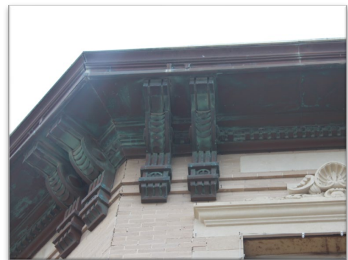
ROOFLINE WITH A METAL CORNICE
