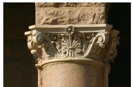
COLUMN CAPITAL OF CUT STONE
