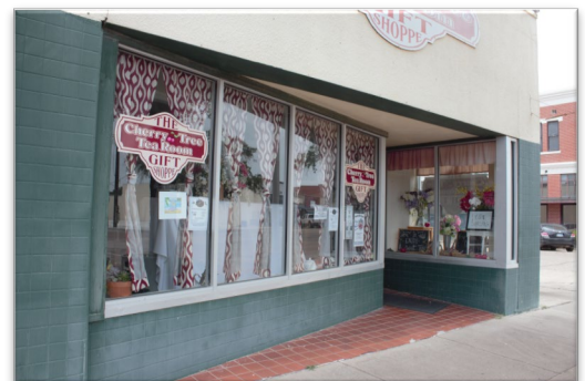
COMMERICAL STOREFRONT WITH RECESSED ENTRANCE AND ANGLED DISPLAY
