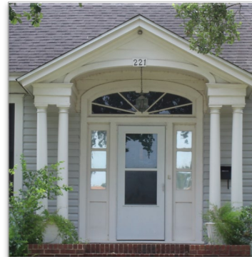
FRONT DOOR WITH SEMI-ELLIPTICAL FANLIGHT AND SIDELIGHTS
