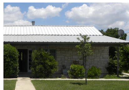
R-PANEL METAL ROOFING
