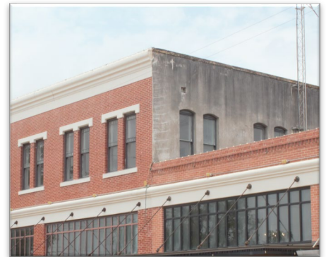
SIMPLE DESIGNS OF SIDE FACADES SHOULD BE MAINTAINED AND NOT “DRESSED” UP
