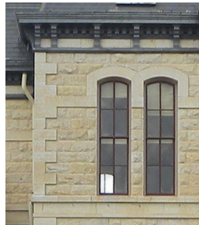
STONE QUOINS ON SIDE OF BUILDING
