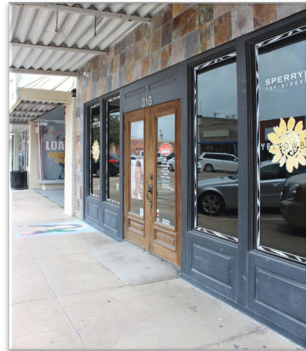
CAST-IRON STOREFRONT ON COMMERCIAL BUILDING
