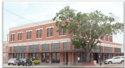
B.O. SIMS BUILDING AT 302 E. KLEBERG AVE.
