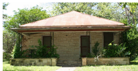
HIP ROOFING ON A HOUSE
