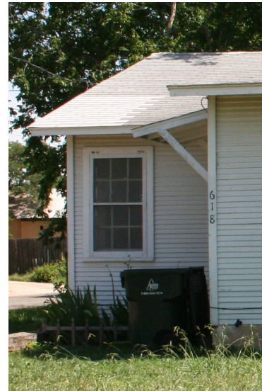
CORNER BOARDS TRIM THE EXTERIOR OF HOUSE
