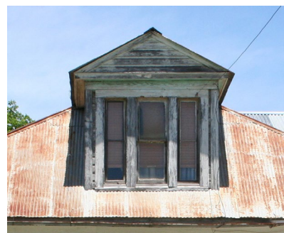
ROOF WITH DORMER PROJECTING OUT
