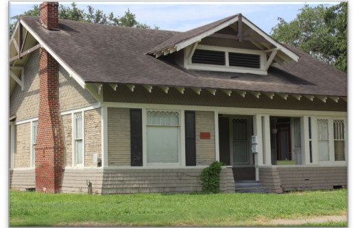
HOUSE WITH MIXED WOOD SHINGLE AND HORIZONTAL WOOD SIDING WITH WOODEN DOOR AND WINDOW SCREENS
