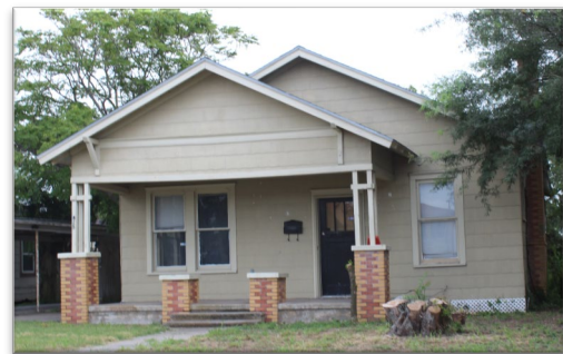
ASBESTOS SHINGLES HAVE BEEN INSTALLED OVER THE ORIGINAL BUILDING MATERIAL OF MANY HOUSES
