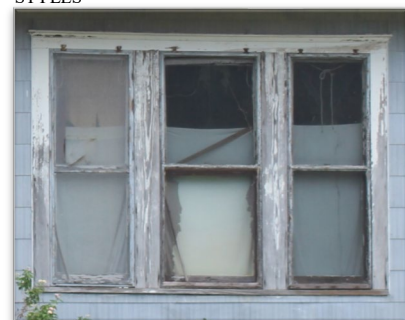
DAMAGED WINDOWS SHOULD BE REPAIRED IN A TIMELY MANNER
