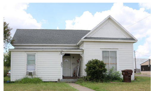
FRONT FACING GABLE ON CROSS GABLE
