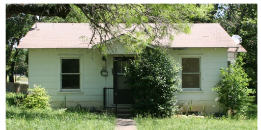
ASBESTOS SHINGLE ON A HOUSE
