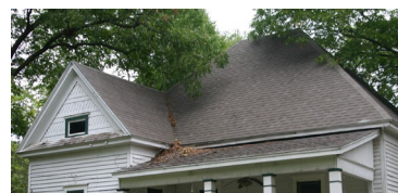
COMBINATION HIP ROOF
