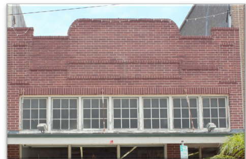
TRANSOM WINDOWS ALLOW LIGHT TO ENTER DEEP INTO THE BUILDING
