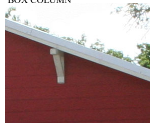
BRACKET UNDER AN EAVE
