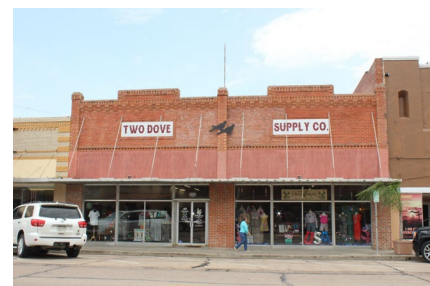
BRICK MASONRY CONSTRUCTION
