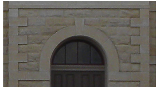
ARCHED HOOD MOULDING OVER WINDOW
