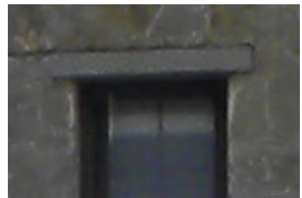
STONE LINTEL OVER WINDOW
