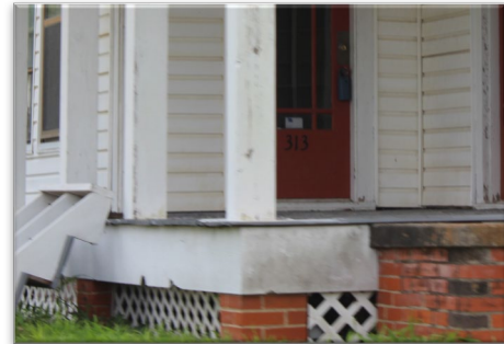
REPLACING THE SKIRTING FROM THE ORIGINAL MATERIAL CHANGES THE APPEARANCE OF THE HOUSE
