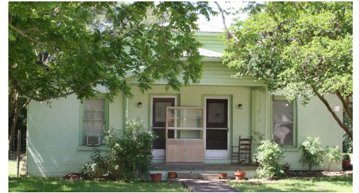
STUCCO CAN RAPIDLY DETERIORATE THE HISTORIC MATERIAL UNDERNEATH AND SHOULD NOT BE INSTALLED
