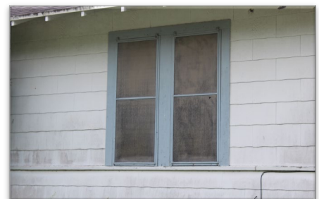
ASBESTOS SIDING ON A HOUSE, BUT WINDOW TRIM REMAINS.
