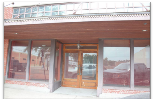
ENTRANCE WITH DOUBLE WOOD DOORS
