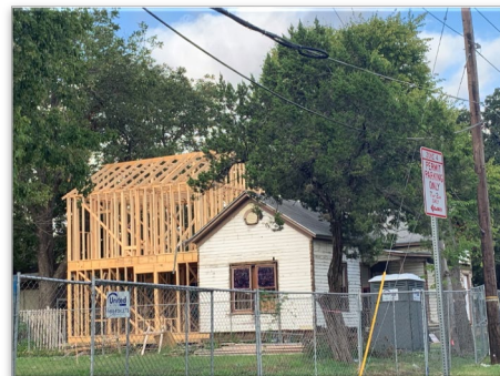
THE ADDITION WILL OVERPOWER THE ORIGINAL HOUSE
