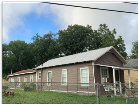
ADDITION AT REAR FOLLOWS WINDOW PATTERN AND DOES NOT COMPETE WITH ORIGINAL
