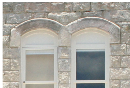
HOOD MOLDING OVER WINDOWS
