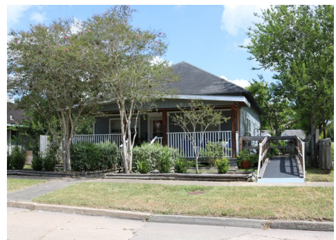
RAMP BUILT TO THE SIDE OF THE HOUSE
