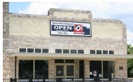
BUILDING WITH TRANSOM WINDOWS
