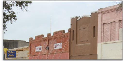
THE ROOFLINE OF A COMMERCIAL BUILDING IS NOT SEEN DUE TO A PARAPET WALL EXTENDING ABOVE IT.
