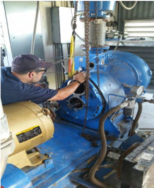
Blower repairs at South treatment plant
