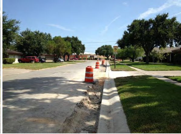
Annette Street drainage improvements
