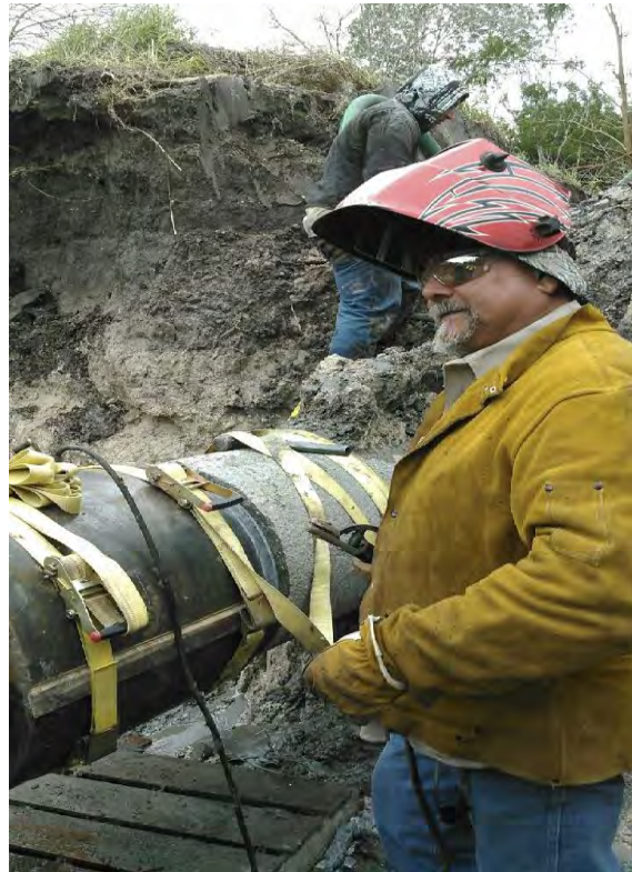
18" water main repair
