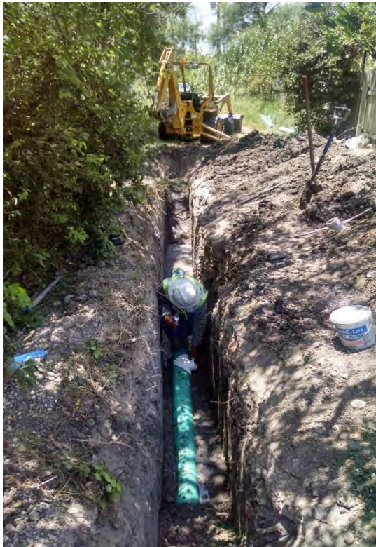
Miller Street sewer line replacement in alley
