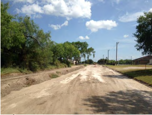
19 th Street reconstruction
