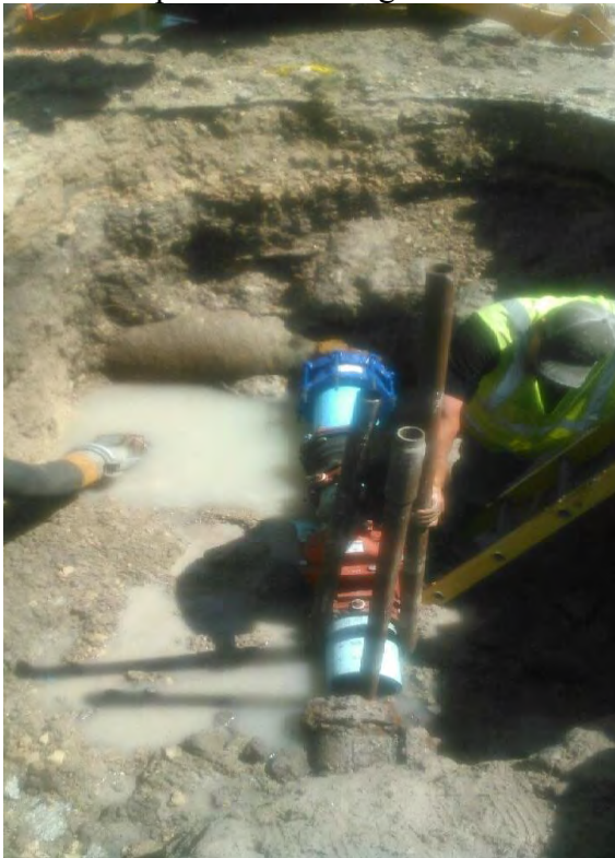
12" water main repair
