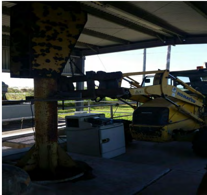
Repairing hoist for UV lights
