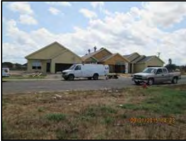
Manuel Buentuello, Building Inspector checking the drip irrigation system at the island along Yoakum Street
