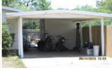
1002 W Kleberg Ave-Junk Warning
