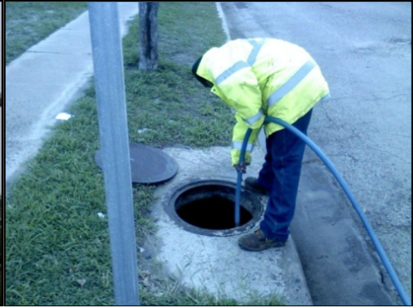
Preparation for Hurricane Season at Santa Gertrudis (cleaning Storm Drain Inlet)
