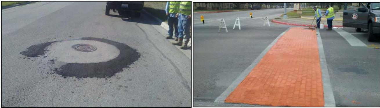
Crews put Cold-mix Asphalt around the manhole at Ailsie between 6<sup>th</sup> and Loop428
