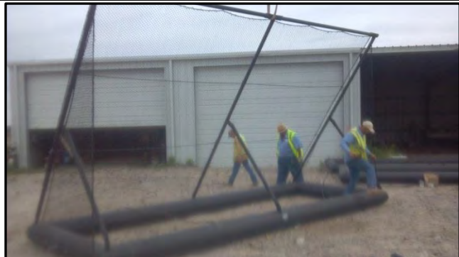
Crews are working on installing new litter Capital Improvement Projects
