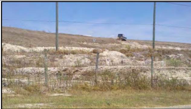
Landfill crews have done grading work to fence Reduce erosion.
