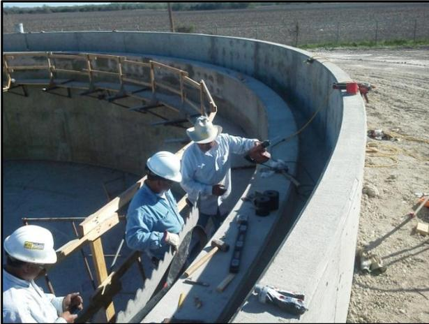
**CSA contractors installing weirs in the clarifier**
