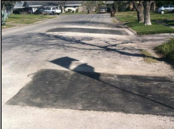
**Street Division has recently purchased a ProPatch machine which uses hot-mix asphalt for patching. Crews cut a square around the pot-hole before filling with hot-mix. The patched area looks nice and it is durable.**
