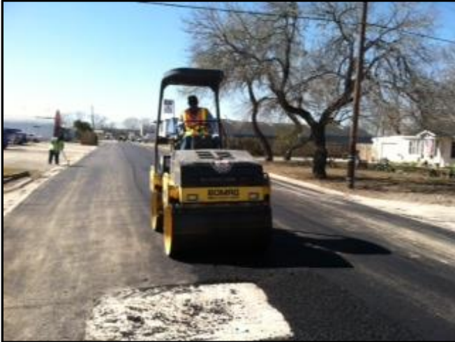
Final compaction on Shelton Street
