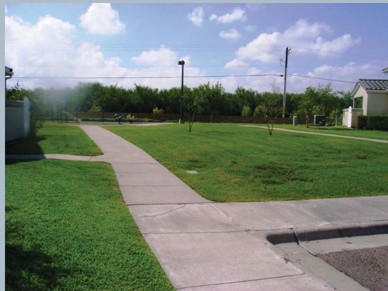
Sidewalks inside a development and along the community's street network can link neighborhoods, parks, schools, and commercial areas.
