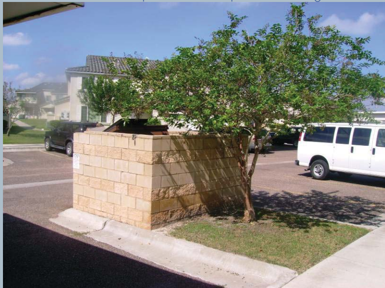
Better screening of parking lots, loading and storage areas, and ground- and building-mounted equipment will improve the appearance of development. This Hunter's Cove example illustrates the shielding of trash containers with quality wall materials and landscaping.
