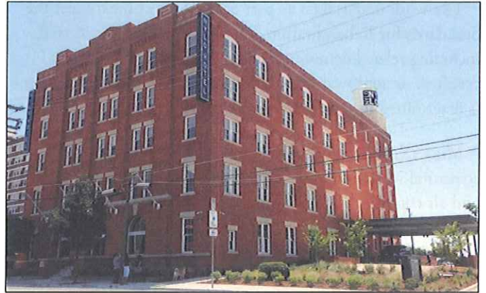
The 1910 building that once housed the Dallas Coffin Company has been rehabilitated into the Nylo Southside Boutique Hotel.
