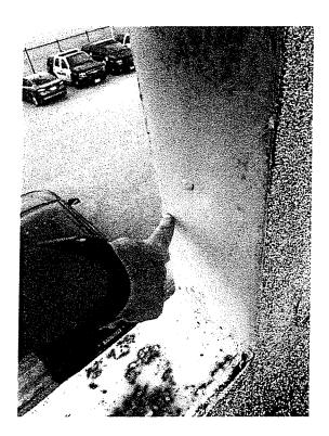
PVC Vinyl Coated Metal scupper insert shall be back sealed and terminated, at 6" oc intervals, around the entire perimeter of the existing scupper metal at the location indicated in the picture.
