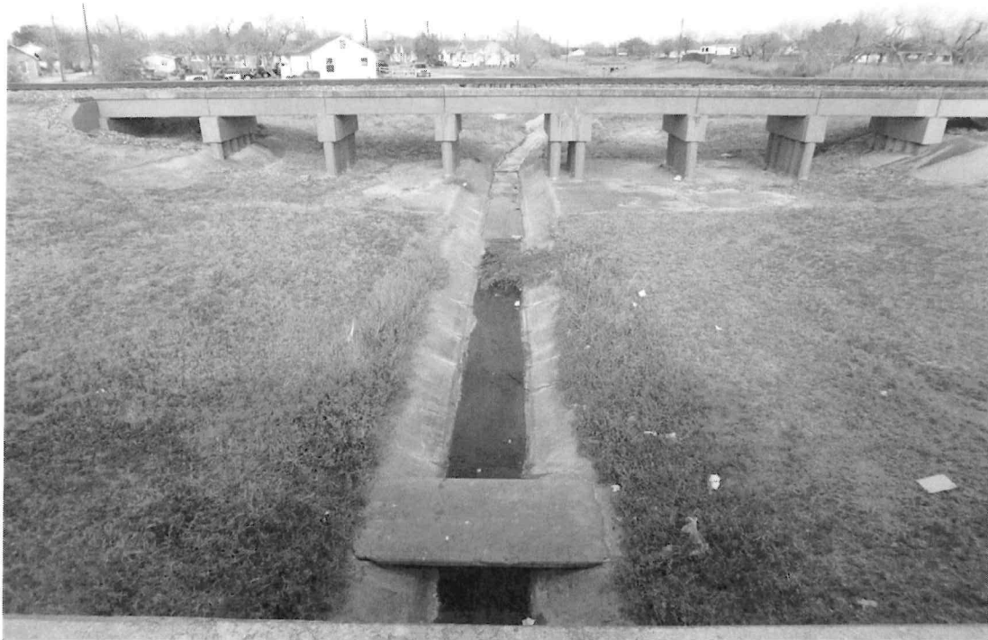
VIEW 5 - UPSTREAM LOOKING WEST
