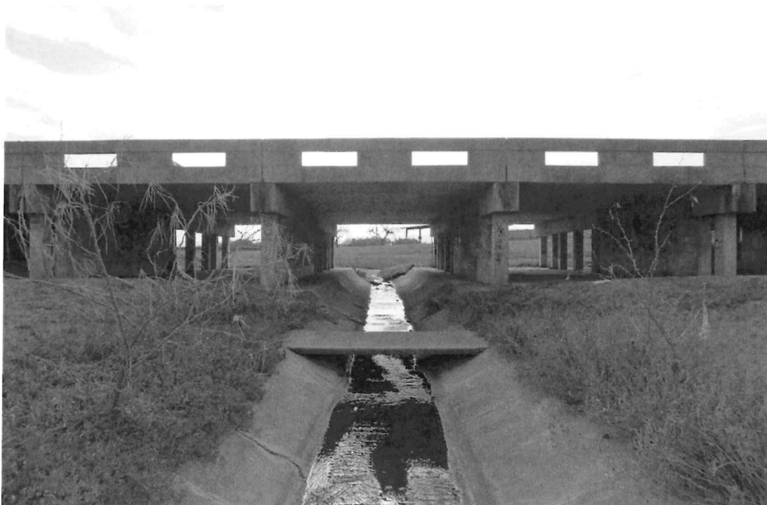
VIEW 4 - STREAM UNDER LOOKING EAST
