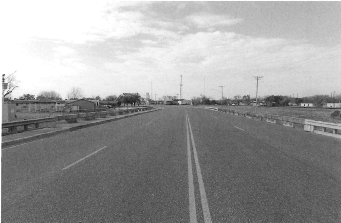
VIEW 1 - ROAD OVER - 6TH STREET LOOKING SOUTH
