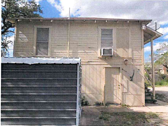
Garage South View
