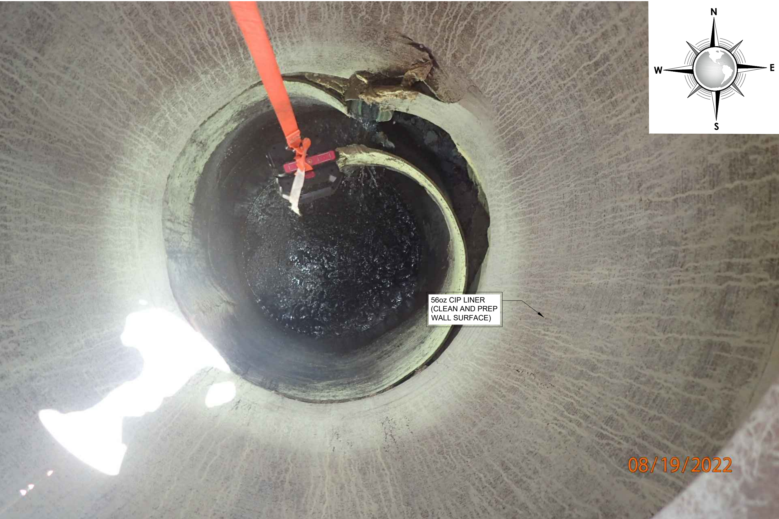
2 C52C52 SANITARY SEWER MANHOLE 52 INTERIOR REHABILITATION PLAN (PHOTO) SCALE : N.T.S.
