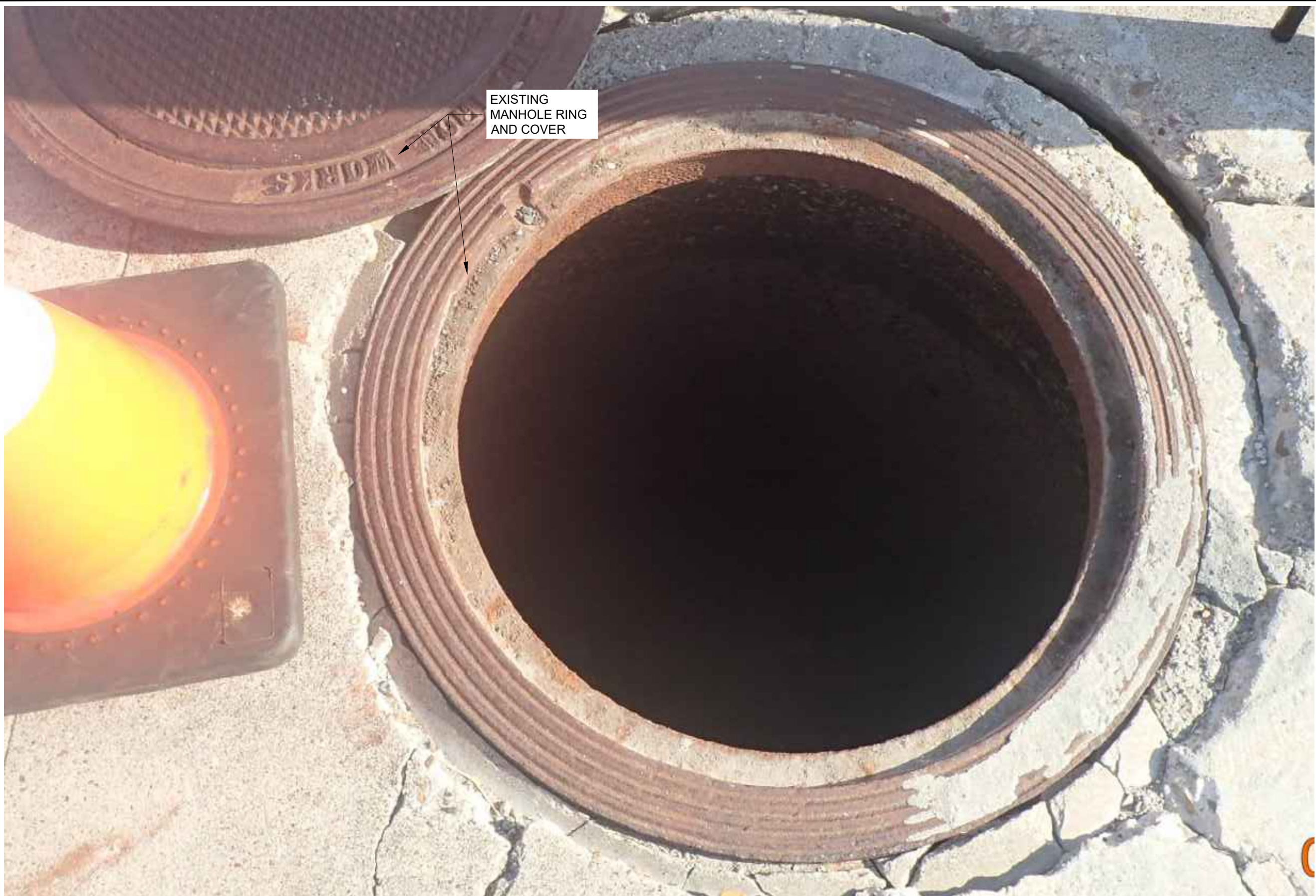
1 SANITARY SEWER MANHOLE 11 EXISTING EXTERIOR REHABILITATION PLAN (PHOTO) C14 C14 SCALE: N.T.S.
