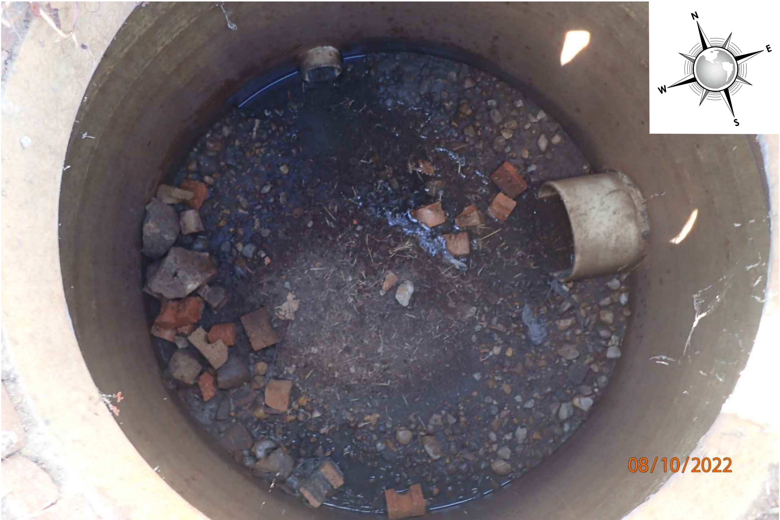
2 C19 C19 SANITARY SEWER MANHOLE 16 INTERIOR REHABILITATION PLAN (PHOTO) SCALE : N.T.S.
