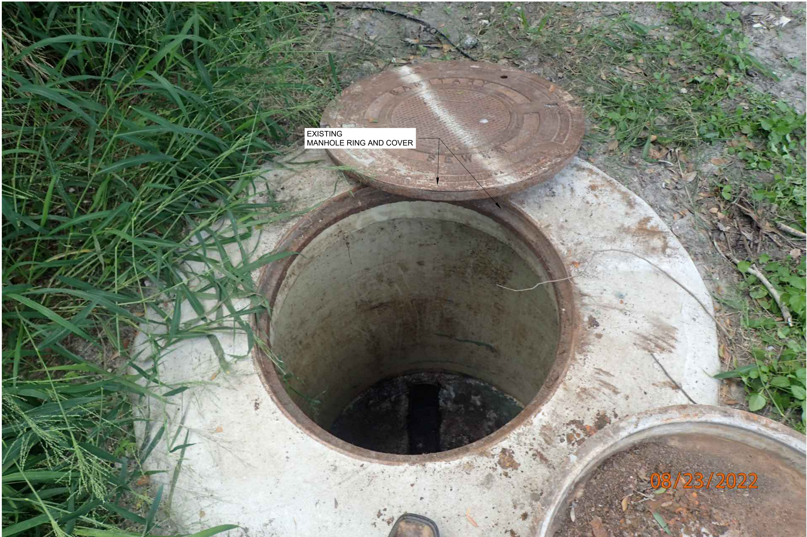
1 C61C61 SANITARY SEWER MANHOLE 61 EXTERIOR REHABILITATION PLAN (PHOTO) SCALE : N.T.S.
