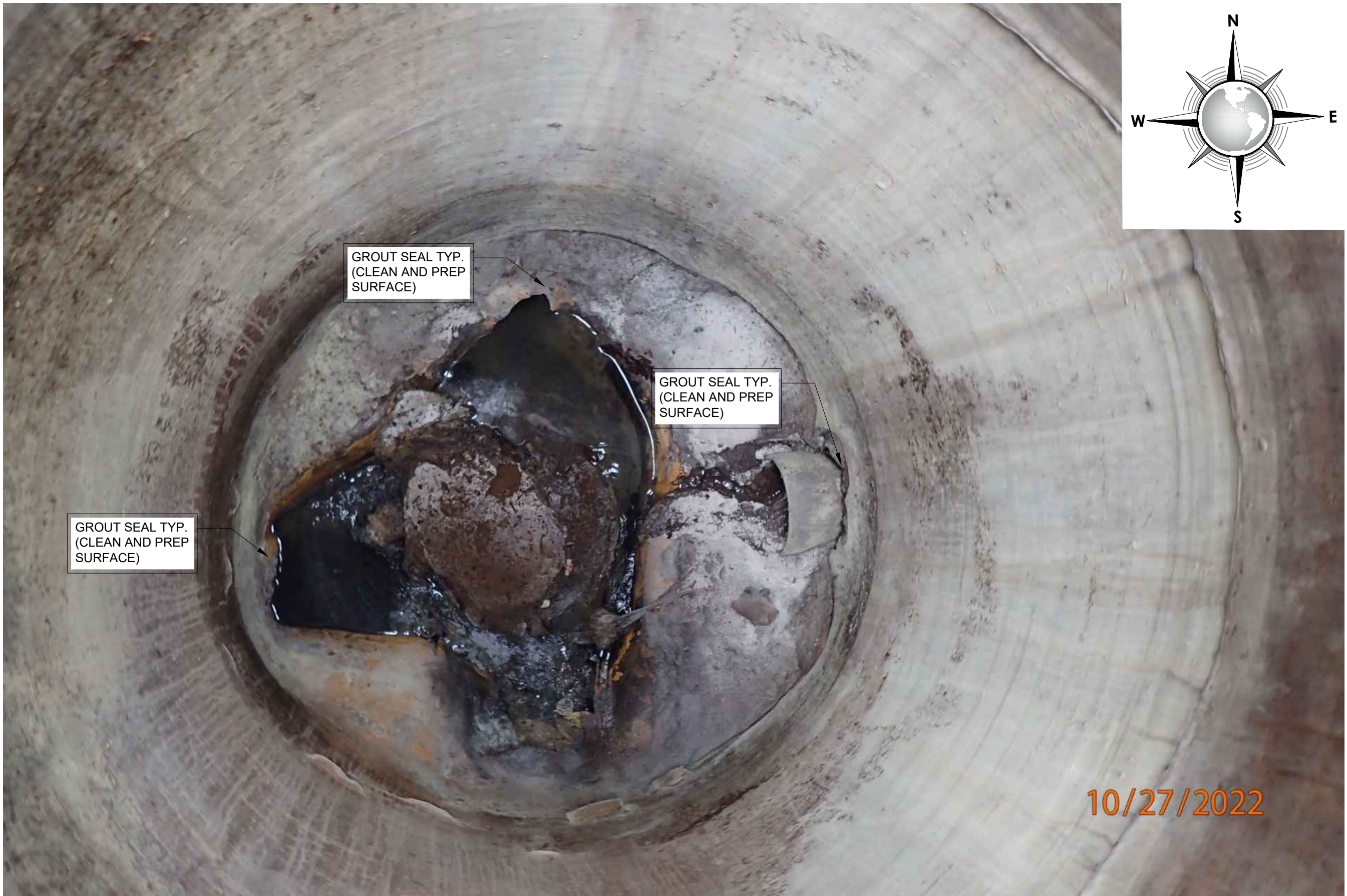
2 SANITARY SEWER MANHOLE 6 INTERIOR REHABILITATION PLAN (PHOTO) SCALE : N.T.S.
