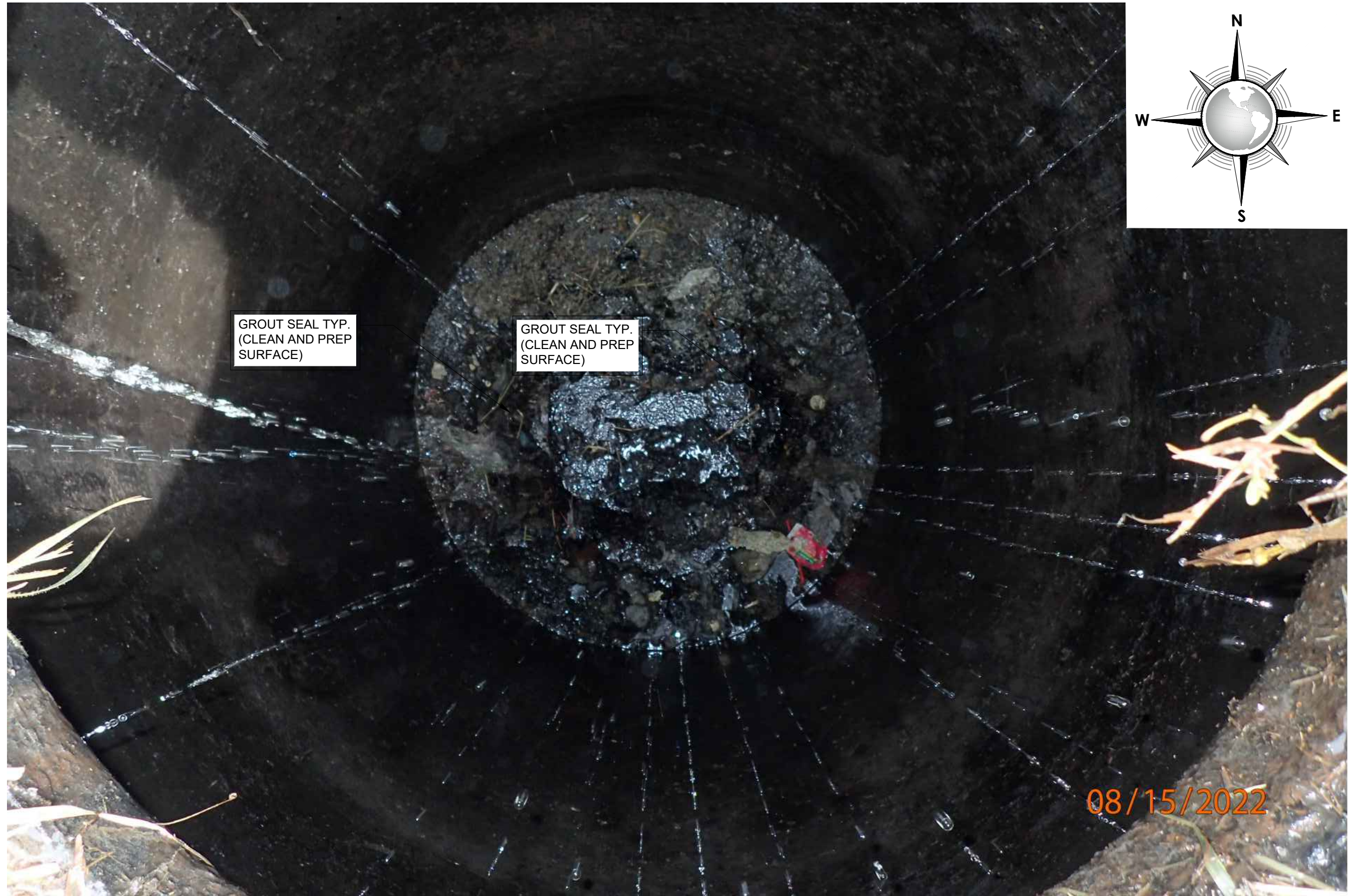
2 C26C26 SANITARY SEWER MANHOLE 24 INTERIOR REHABILITATION PLAN (PHOTO) SCALE : N.T.S.
