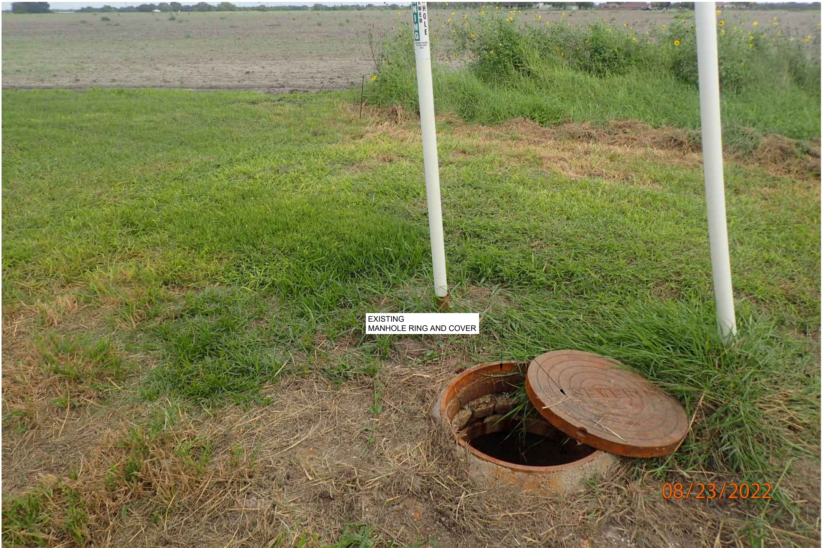
1 C60C60 SANITARY SEWER MANHOLE 60 EXTERIOR REHABILITATION PLAN (PHOTO) SCALE : N.T.S.
