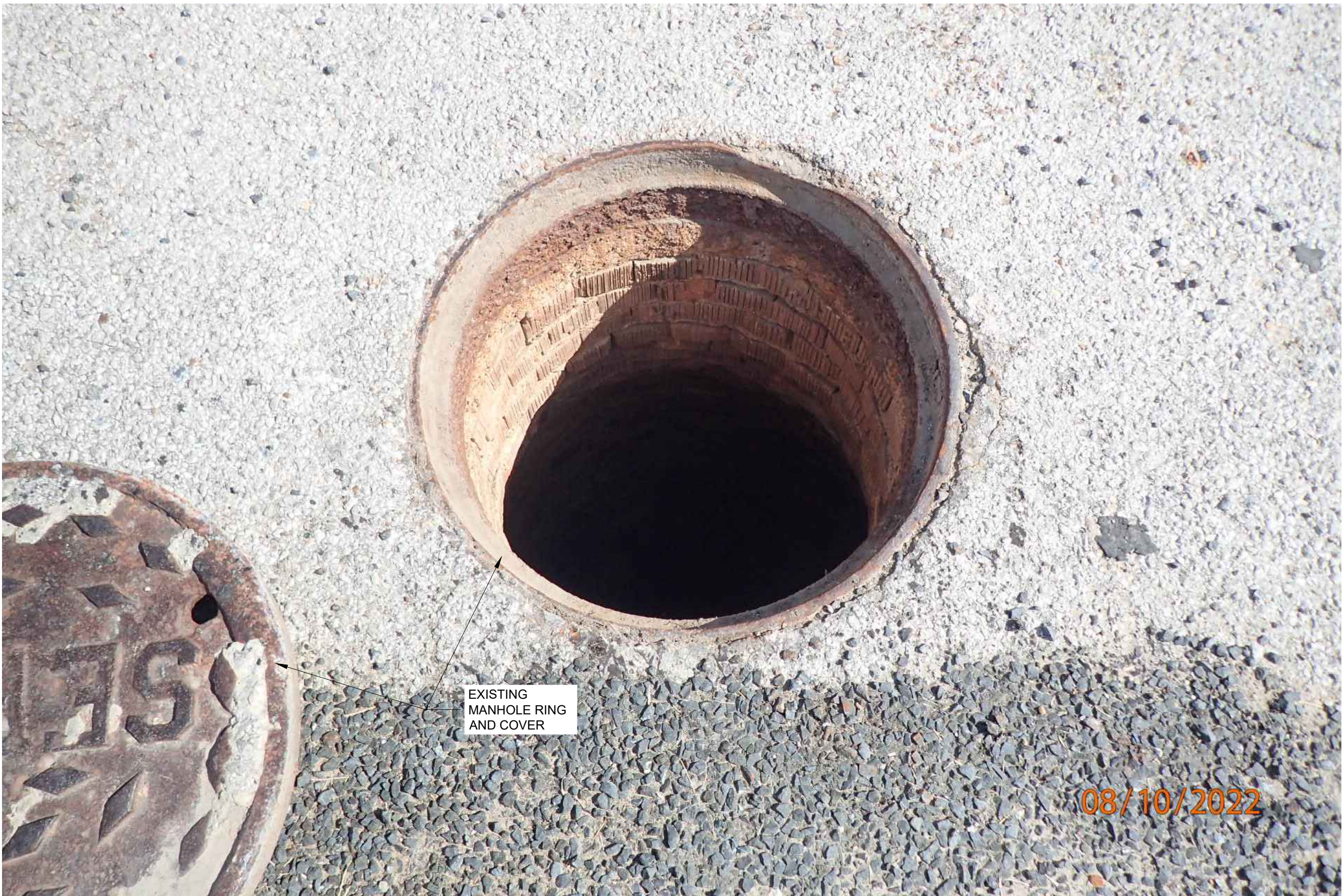
1 C15C15 SANITARY SEWER MANHOLE 12 EXISTING EXTERIOR REHABILITATION PLAN (PHOTO) SCALE : N.T.S.
