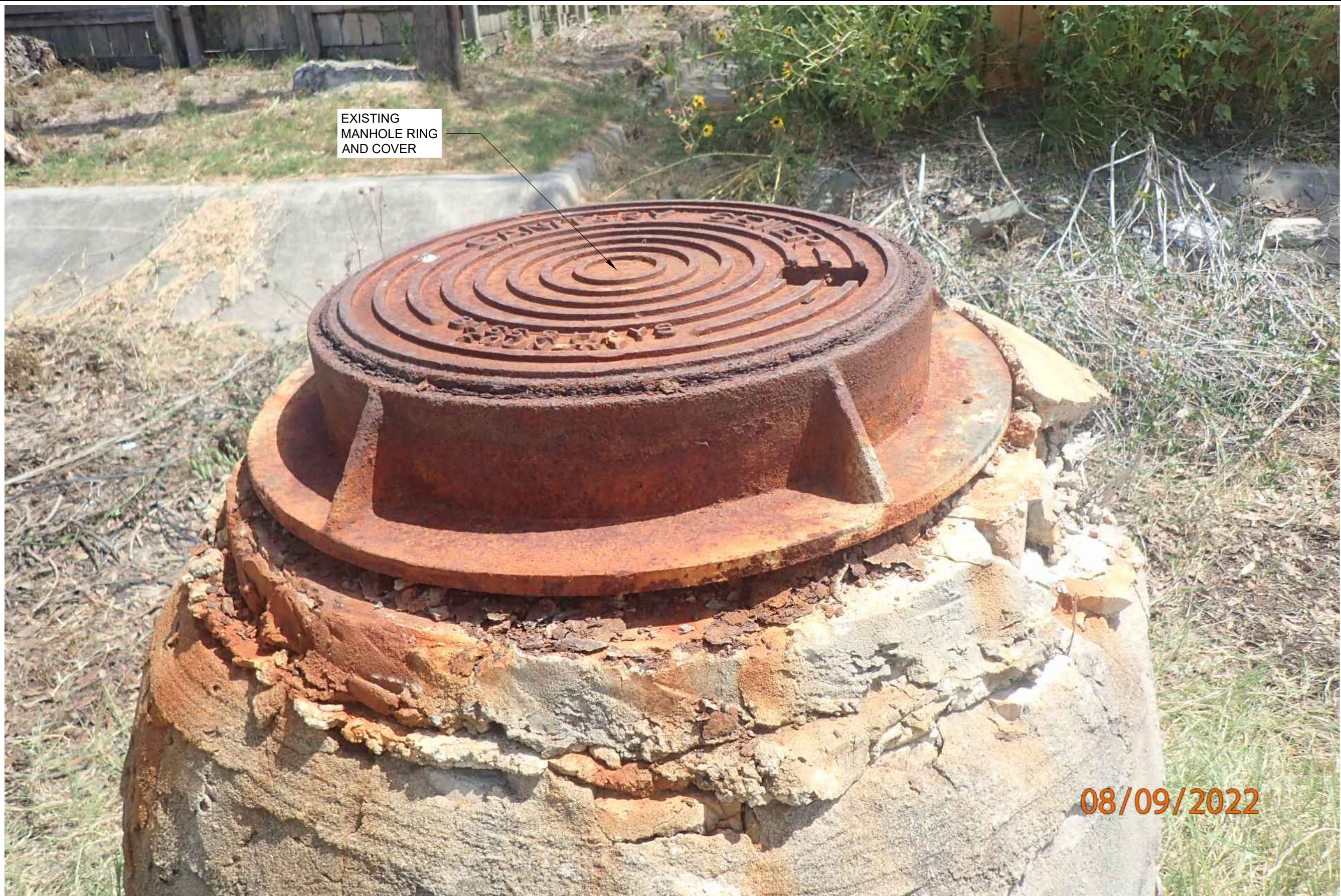
1 SANITARY SEWER MANHOLE 6 EXTERIOR REHABILITATION PLAN (PHOTO) SCALE : N.T.S.
