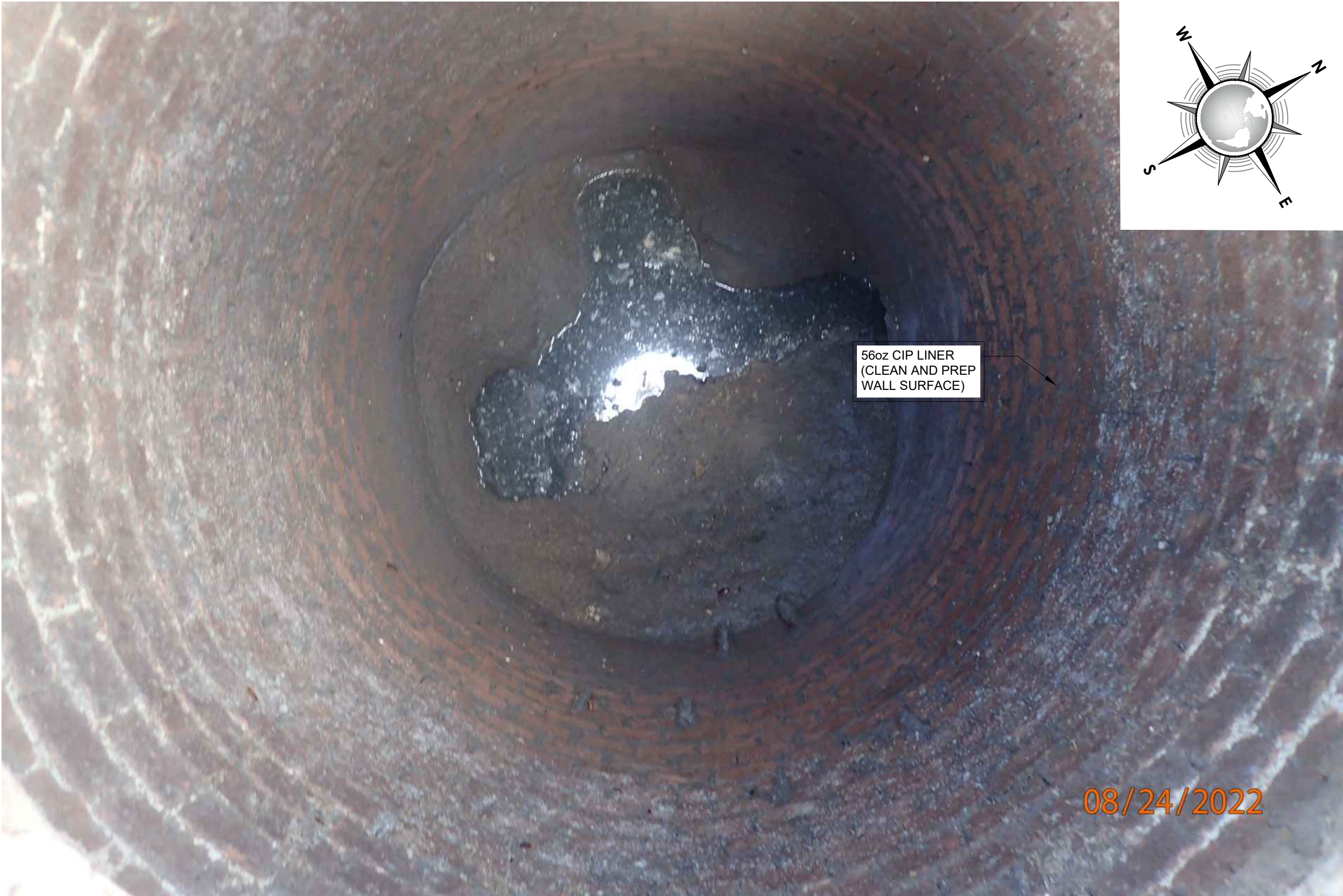
2 C68C68 SANITARY SEWER MANHOLE 68 INTERIOR REHABILITATION PLAN (PHOTO) SCALE : N.T.S.
