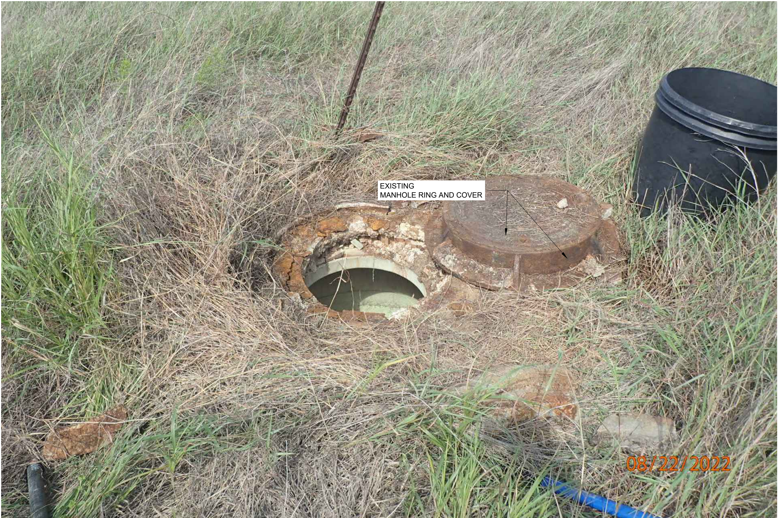
1 C55C55 SANITARY SEWER MANHOLE 55 EXTERIOR REHABILITATION PLAN (PHOTO) SCALE : N.T.S.
