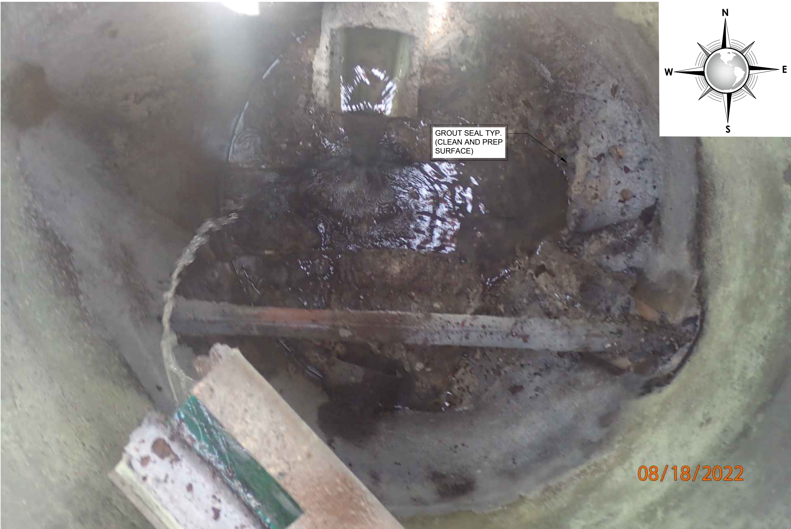
2 C47C47 SANITARY SEWER MANHOLE 47 INTERIOR REHABILITATION PLAN (PHOTO) SCALE : N.T.S.
