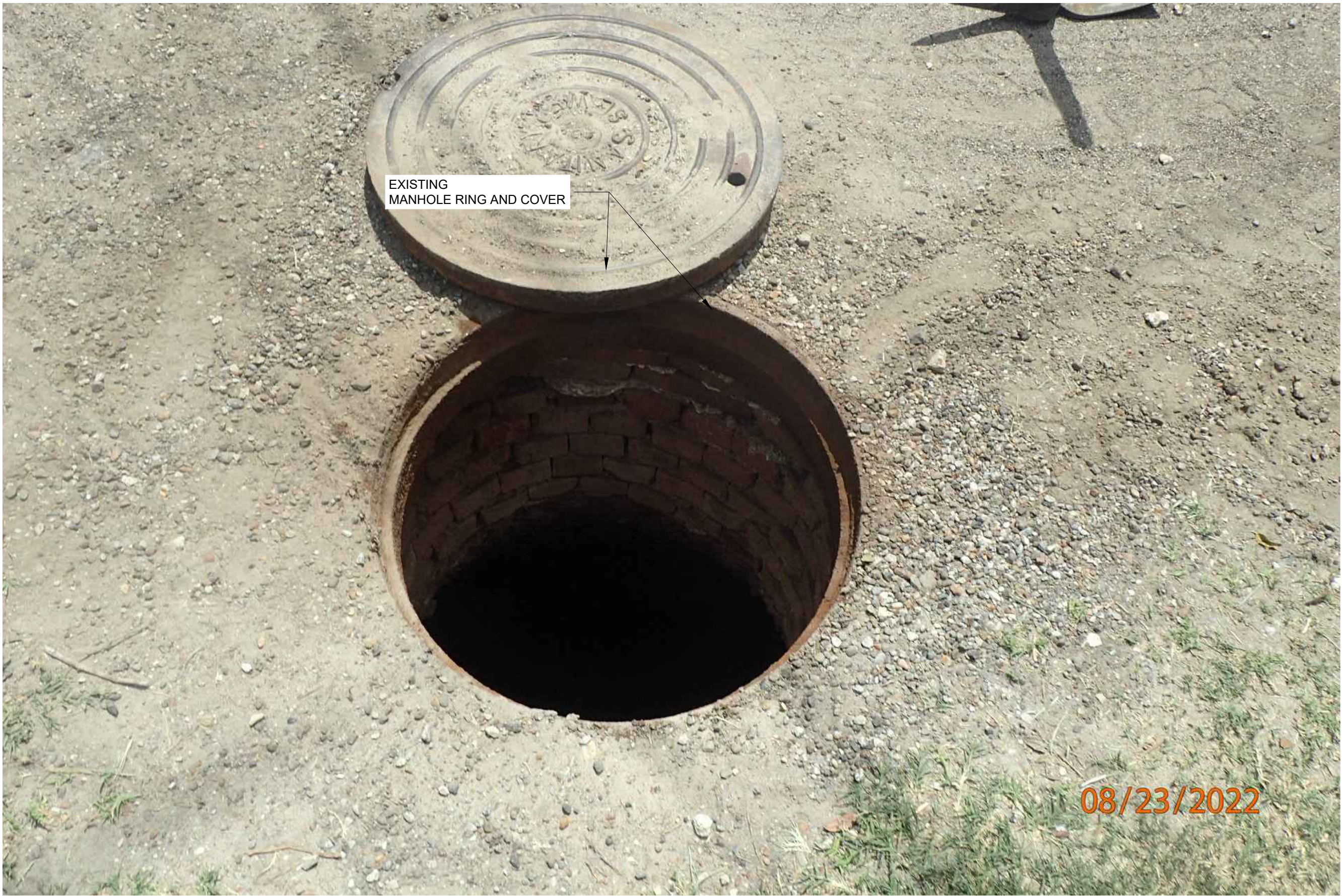
1 SANITARY SEWER MANHOLE 64 EXTERIOR REHABILITATION PLAN (PHOTO) C64 C64 SCALE : N.T.S.
