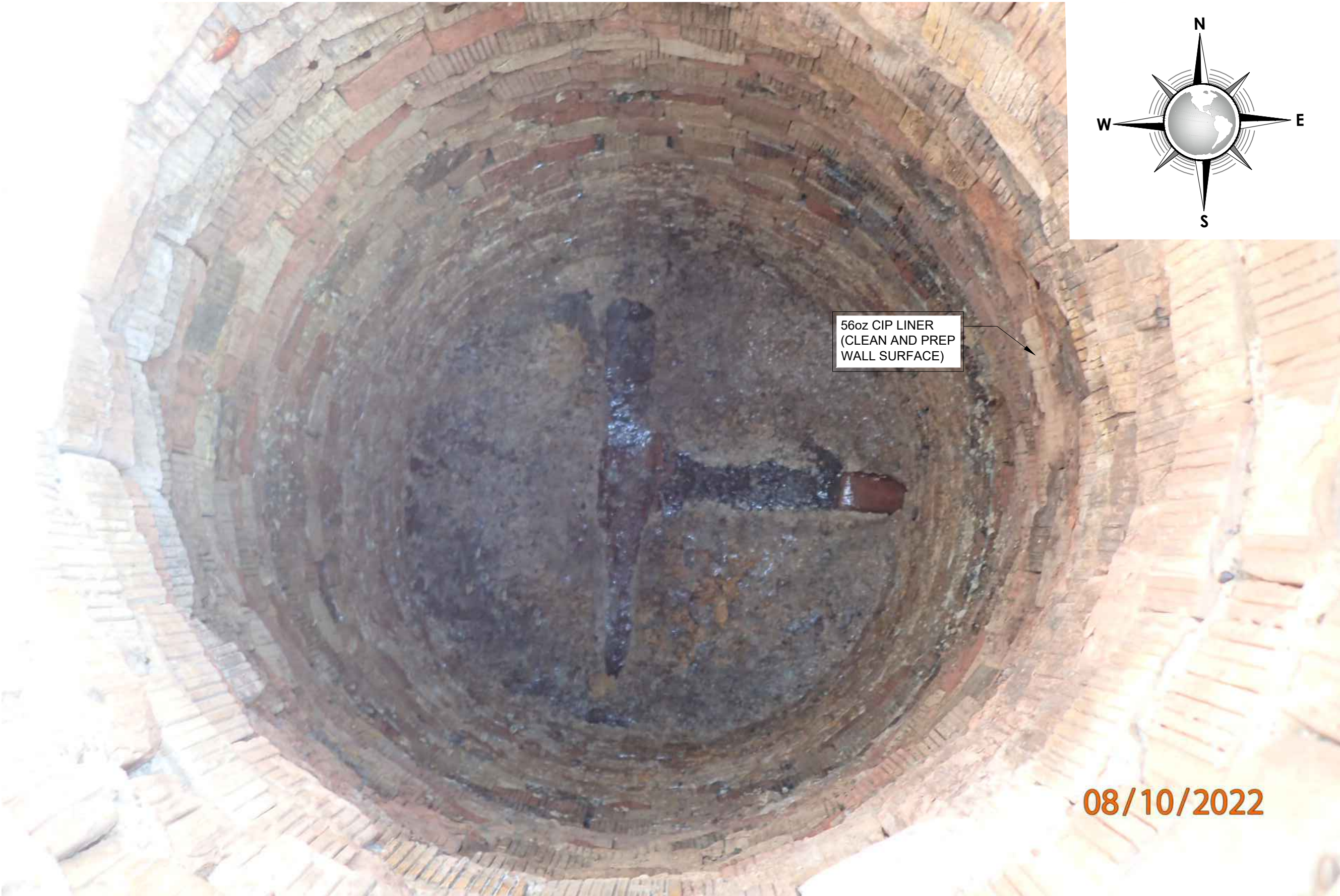
2 C15C15 SANITARY SEWER MANHOLE 12 INTERIOR REHABILITATION PLAN (PHOTO) SCALE : N.T.S.
