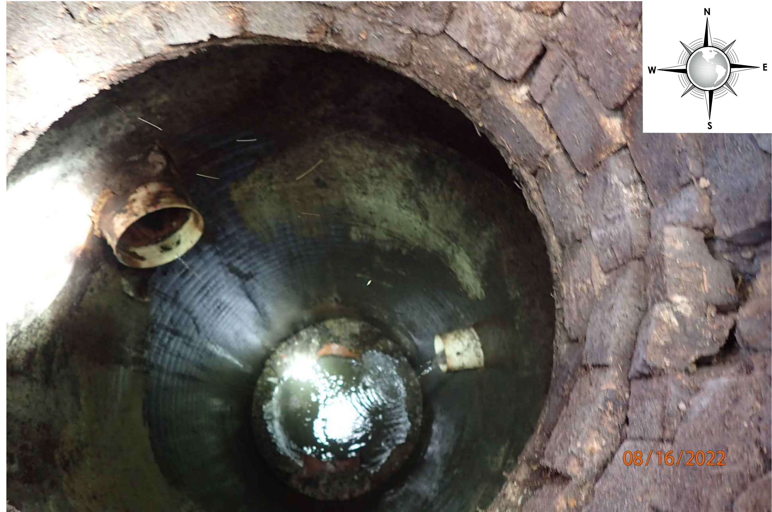
2 C28 C28 SANITARY SEWER MANHOLE 28 INTERIOR REHABILITATION PLAN (PHOTO) SCALE : N.T.S.
