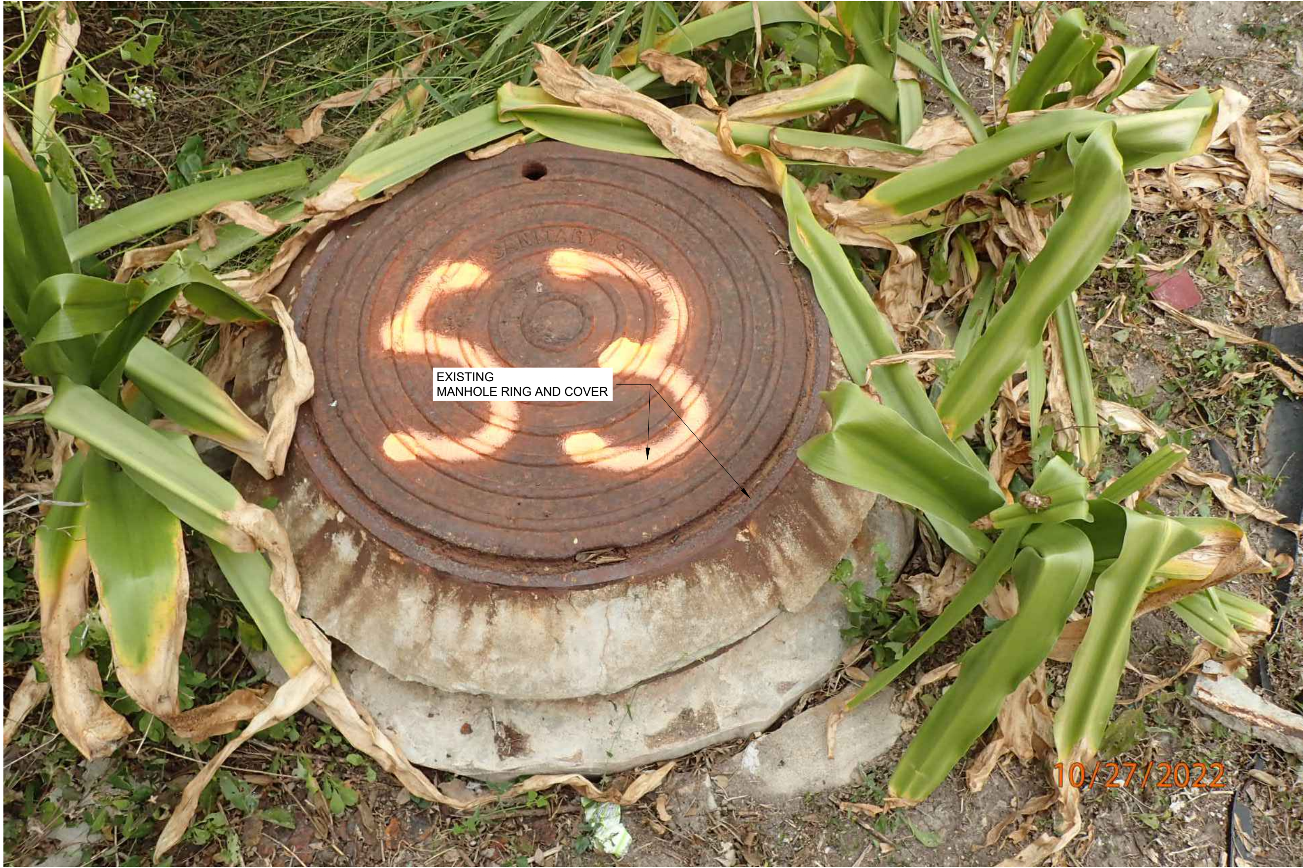
1 C53C53 SANITARY SEWER MANHOLE 53 EXTERIOR REHABILITATION PLAN (PHOTO) SCALE : N.T.S.
