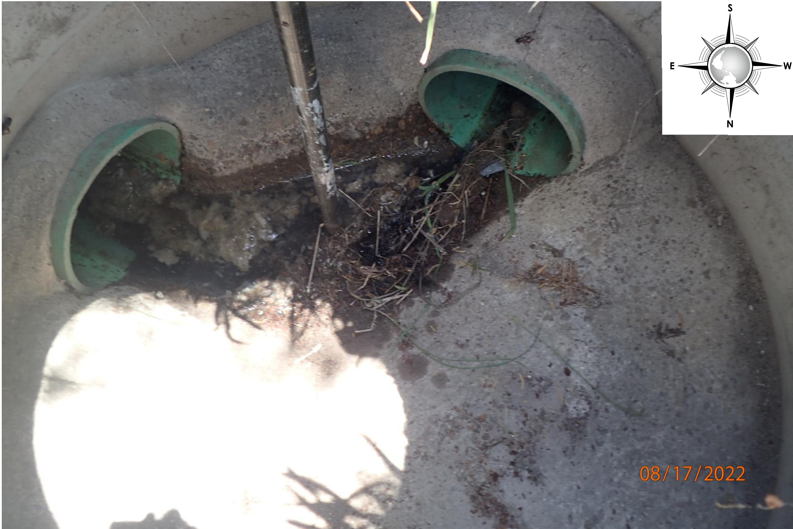
2 C38C38 SANITARY SEWER MANHOLE 38 INTERIOR REHABILITATION PLAN (PHOTO) SCALE : N.T.S.
