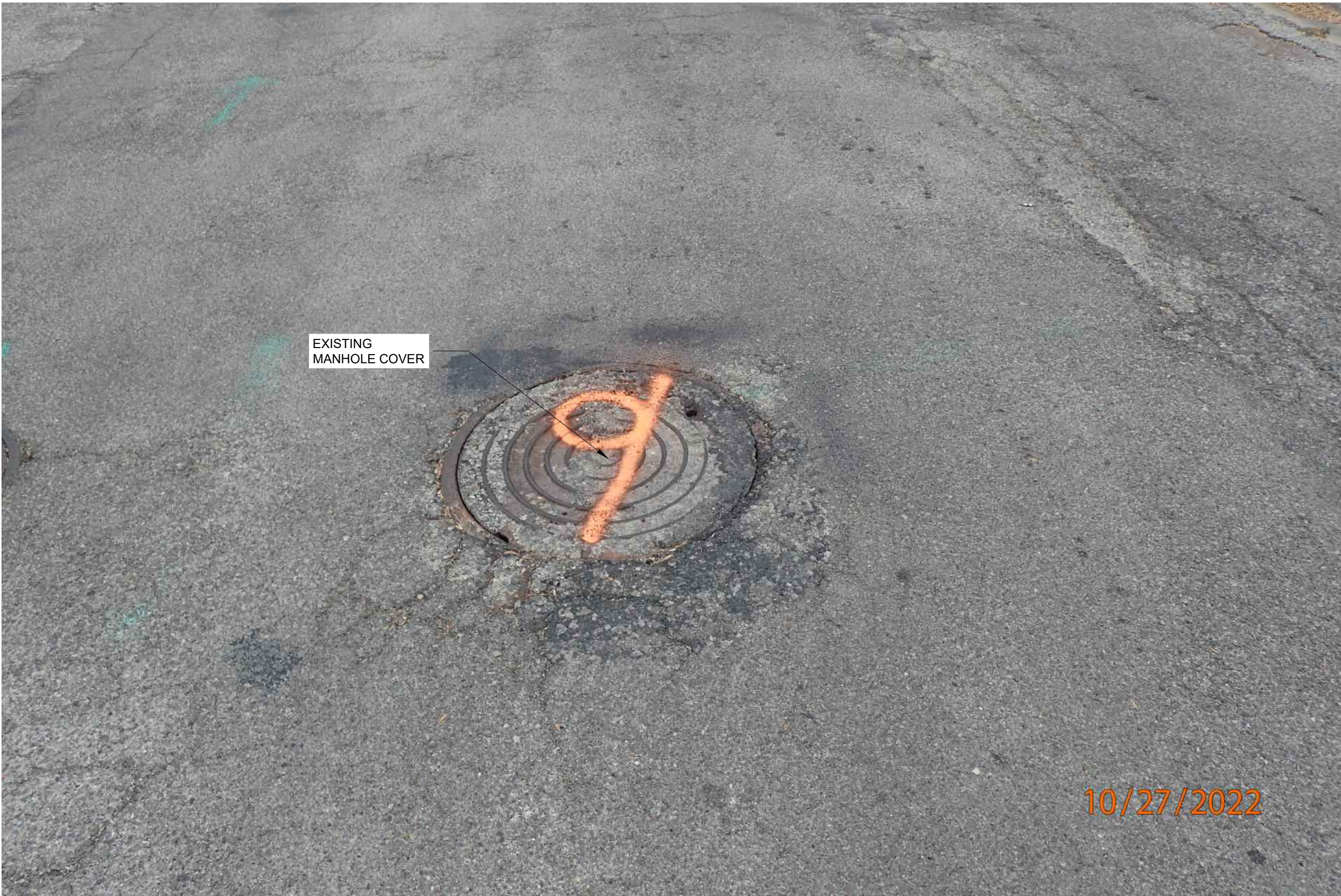
1 C12 C12 SANITARY SEWER MANHOLE 9 EXISTING EXTERIOR REHABILITATION PLAN (PHOTO) SCALE : N.T.S.
