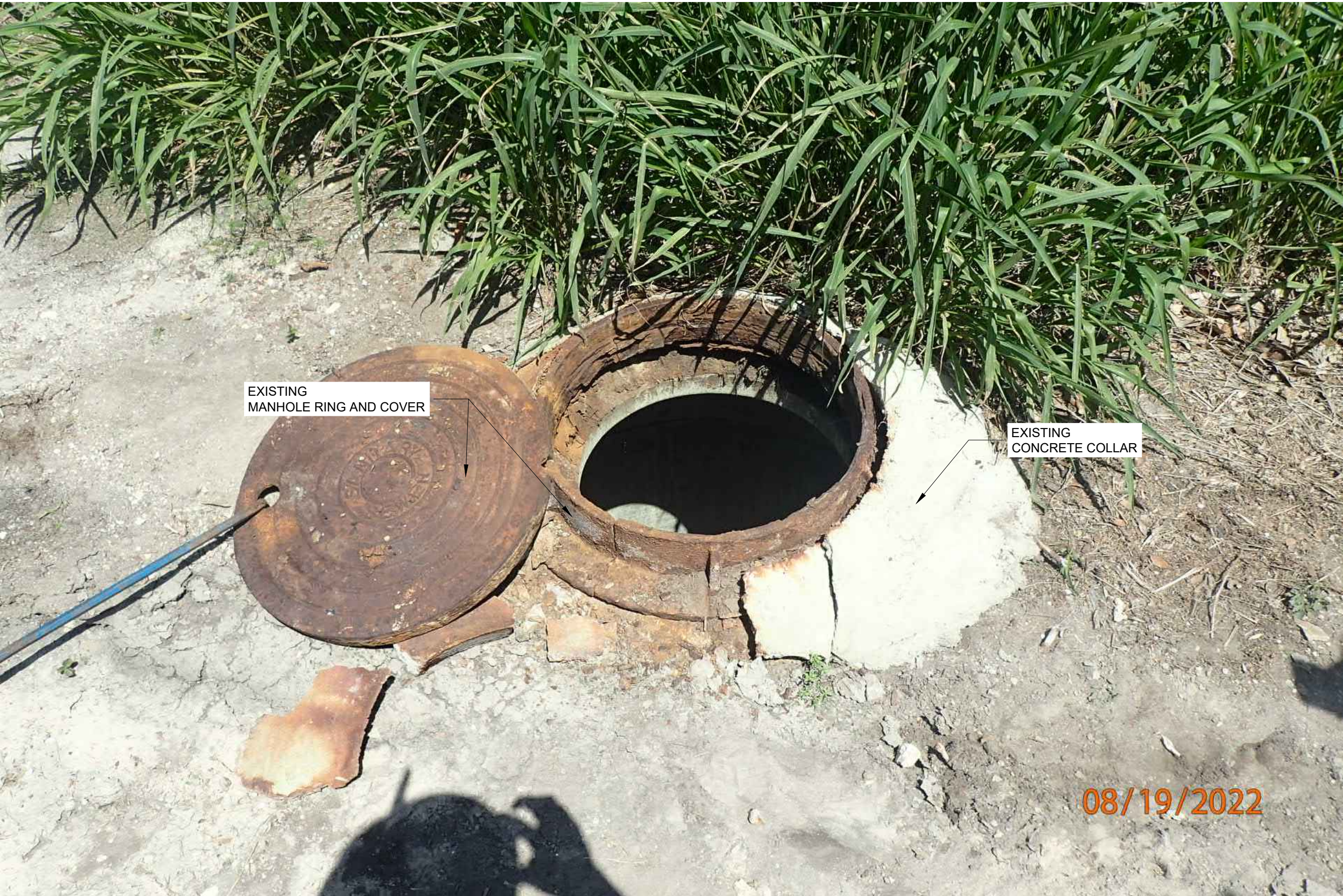
1 C52C52 SANITARY SEWER MANHOLE 52 EXTERIOR REHABILITATION PLAN (PHOTO) SCALE : N.T.S.
