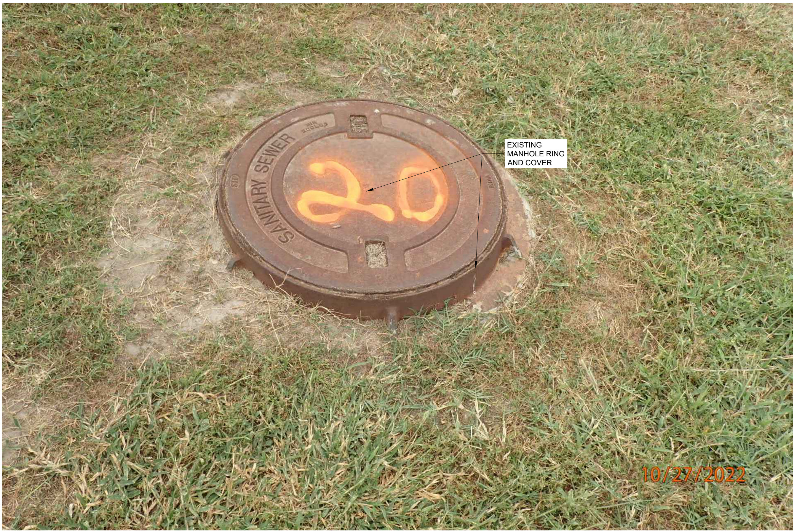
1 C22 C22 SANITARY SEWER MANHOLE 20 EXTERIOR REHABILITATION PLAN (PHOTO) SCALE : N.T.S.
