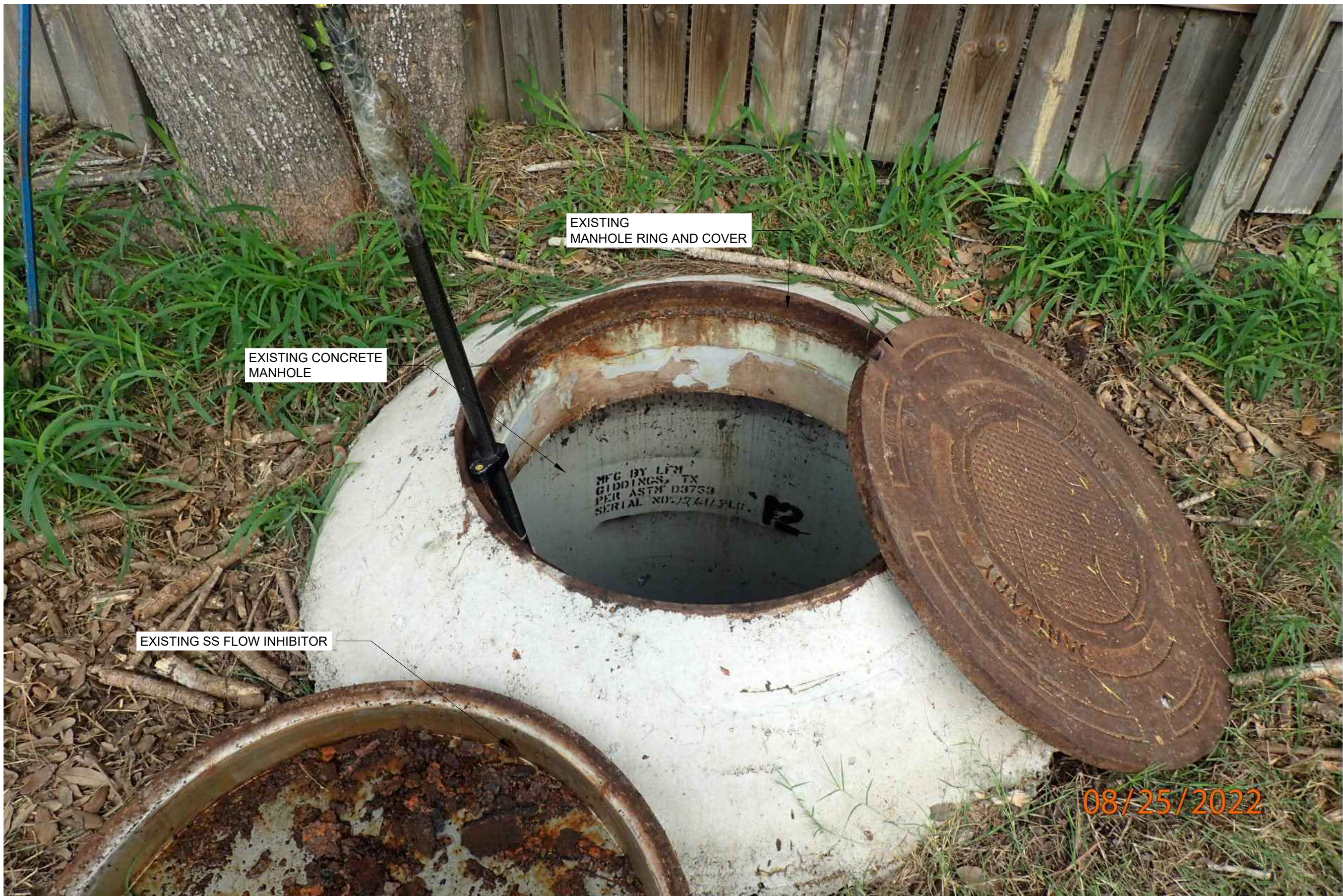
1 C72 C72 SANITARY SEWER MANHOLE 72 EXTERIOR REHABILITATION PLAN (PHOTO) SCALE : N.T.S.
