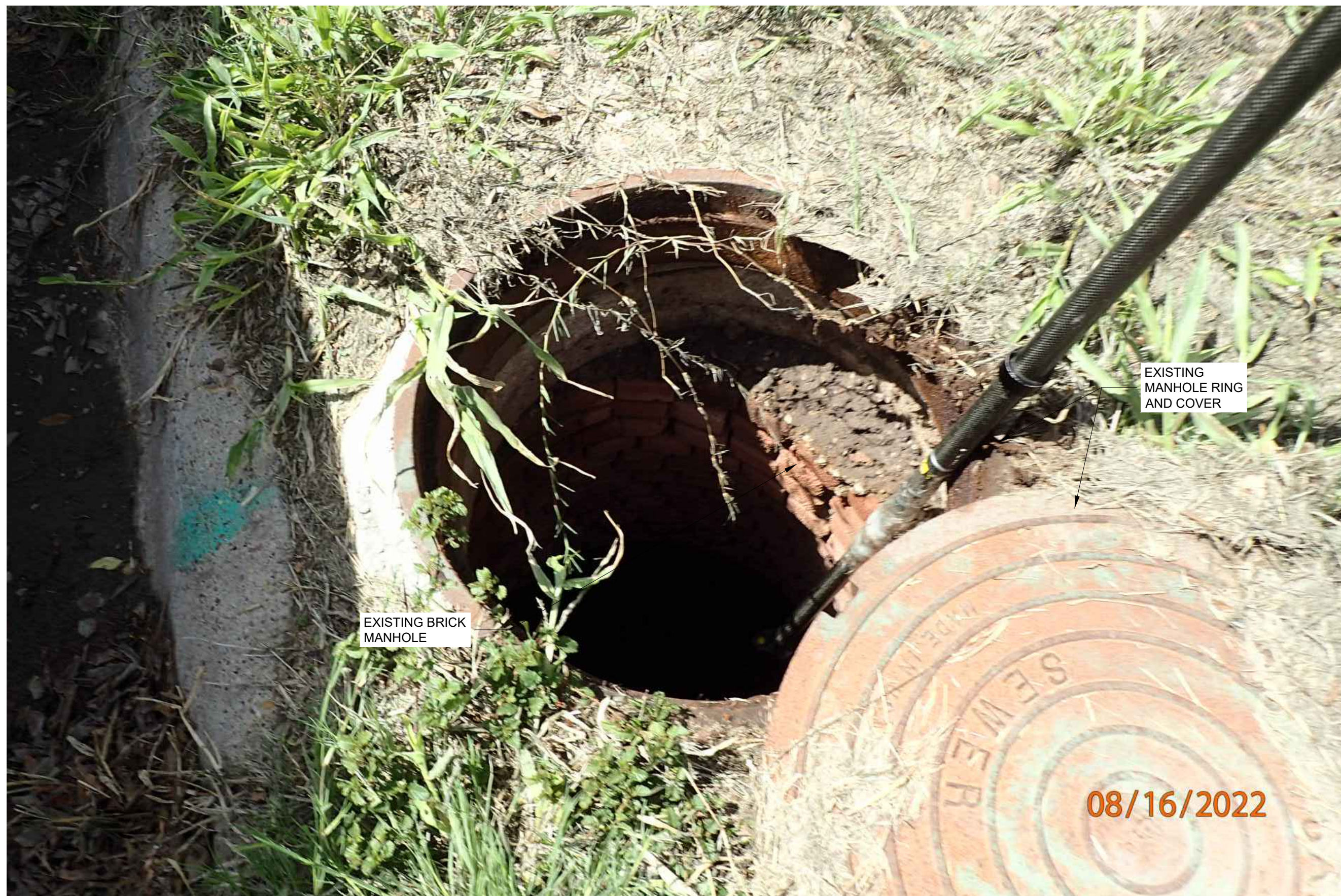
1 SANITARY SEWER MANHOLE 30 EXISTING EXTERIOR REHABILITATION PLAN (PHOTO)
