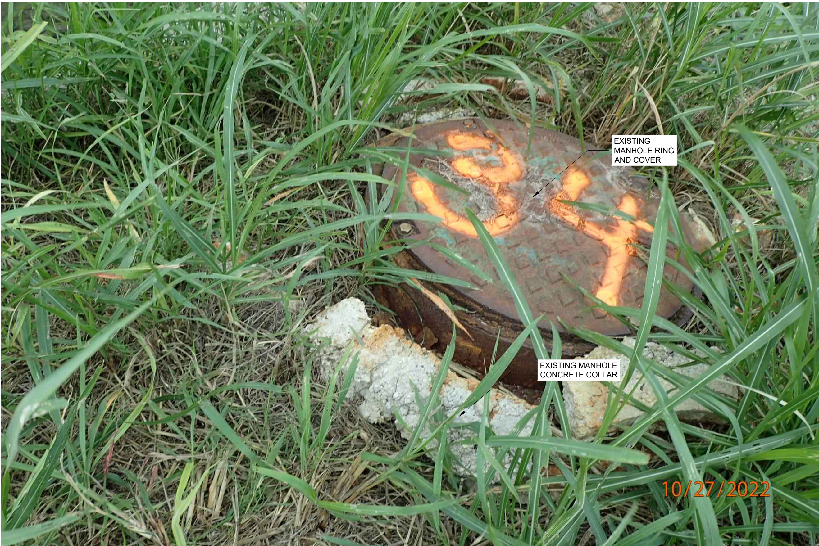
1 SANITARY SEWER MANHOLE 34 EXTERIOR REHABILITATION PLAN (PHOTO) C34 C34 SCALE: N.T.S.
