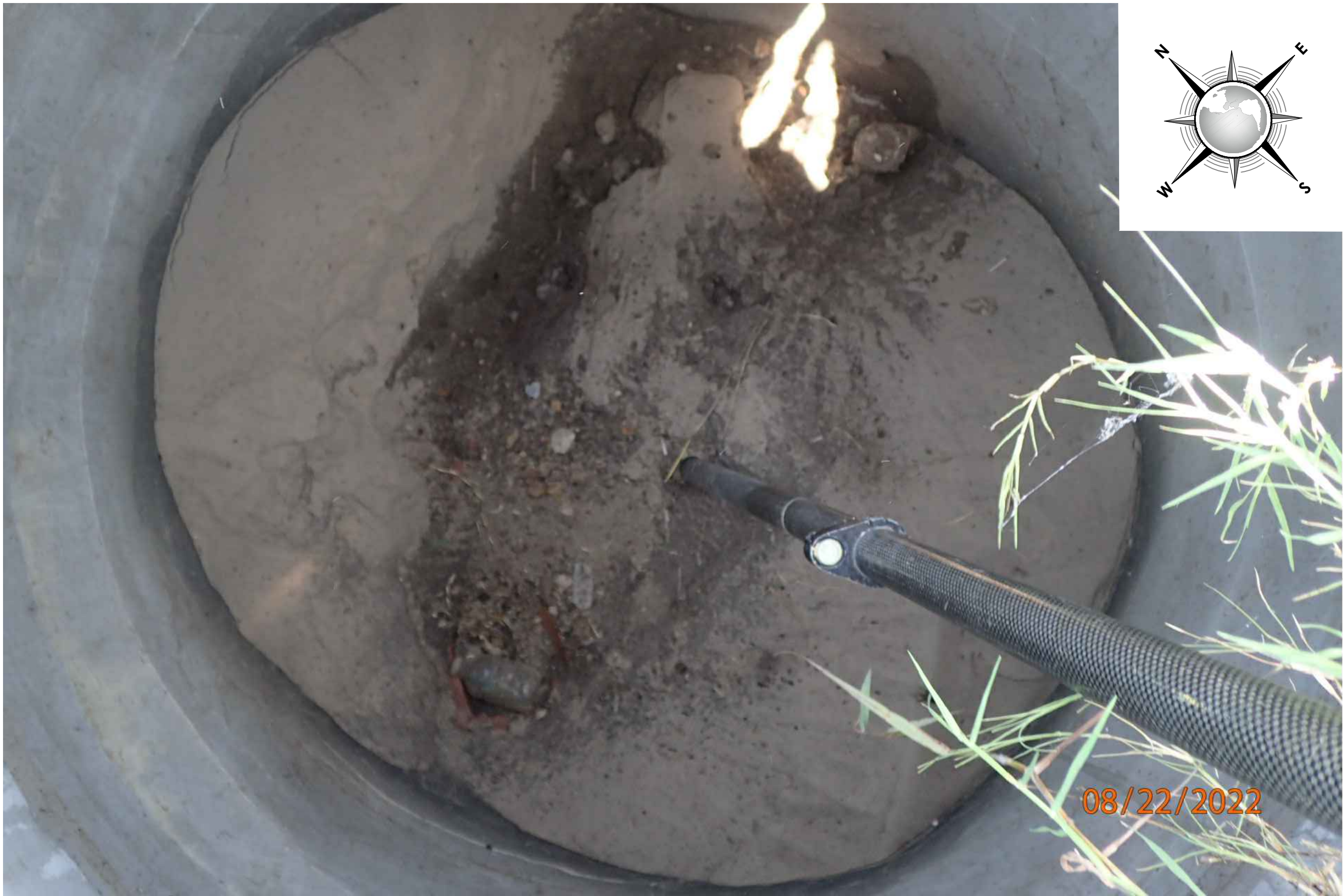
2 C58C58 SANITARY SEWER MANHOLE 58 INTERIOR REHABILITATION PLAN (PHOTO) SCALE : N.T.S.
