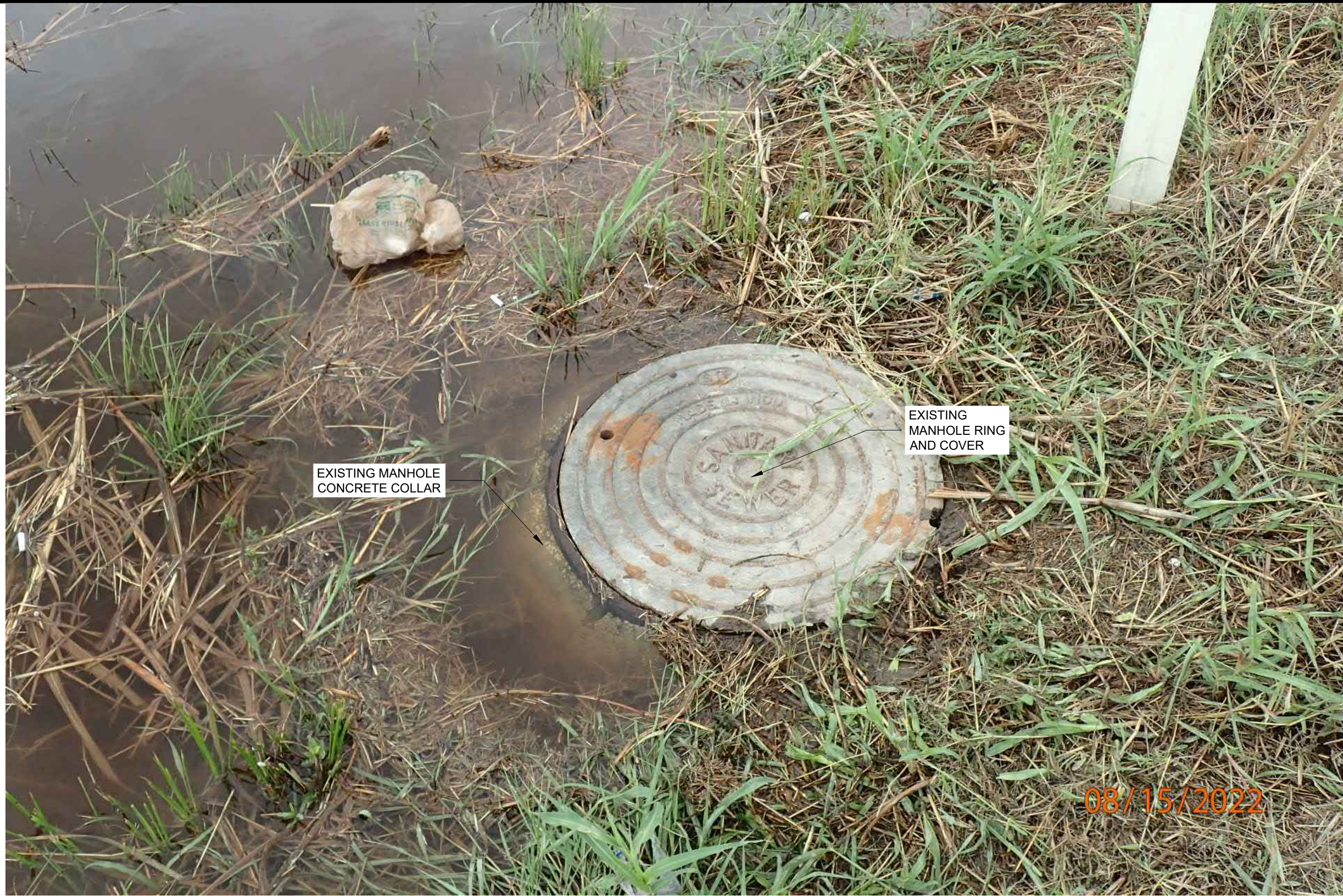
1 C26C26 SANITARY SEWER MANHOLE 24 EXTERIOR REHABILITATION PLAN (PHOTO) SCALE : N.T.S.
