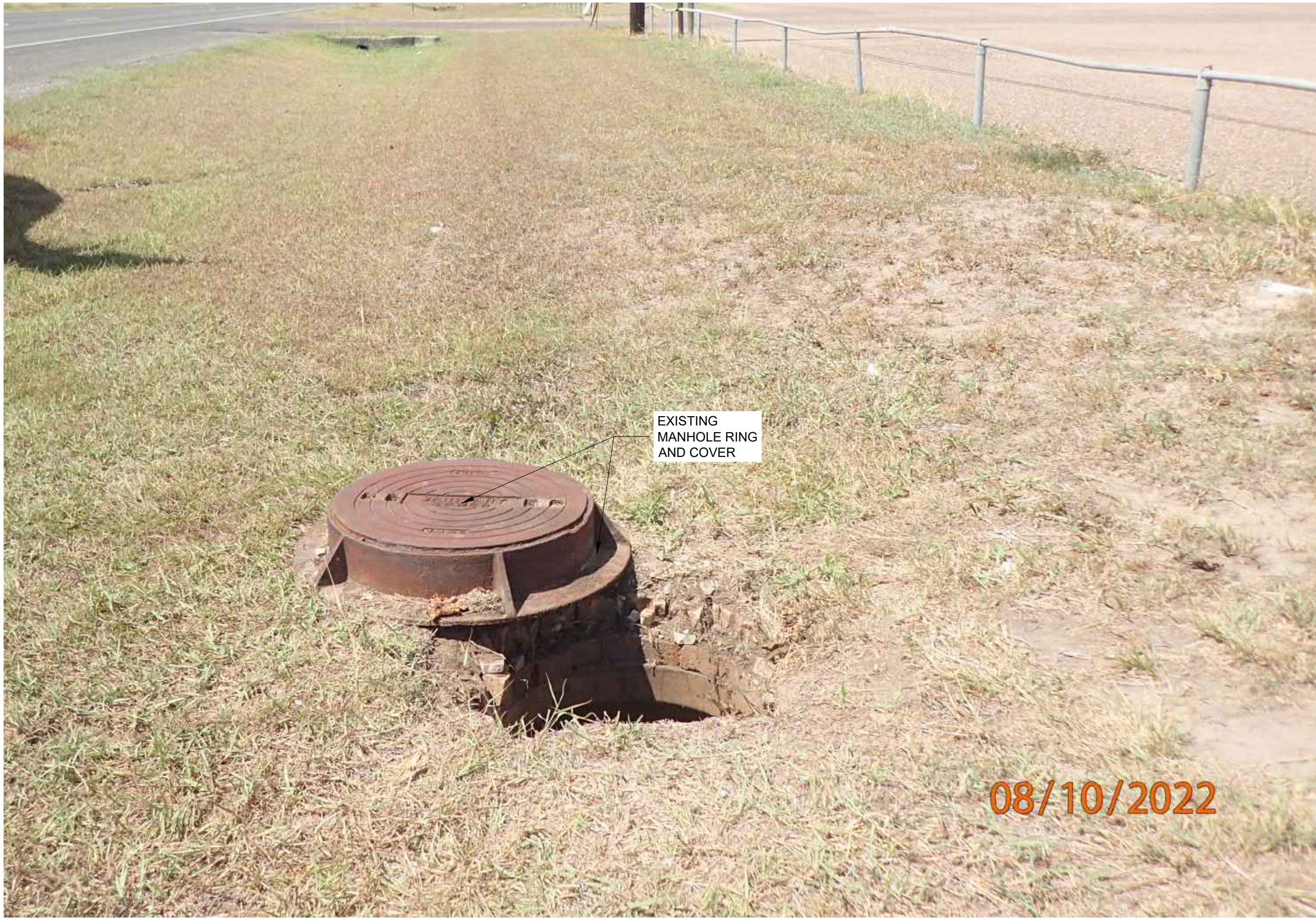
1 C19 C19 SANITARY SEWER MANHOLE 16 EXTERIOR REHABILITATION PLAN (PHOTO) SCALE : N.T.S.
