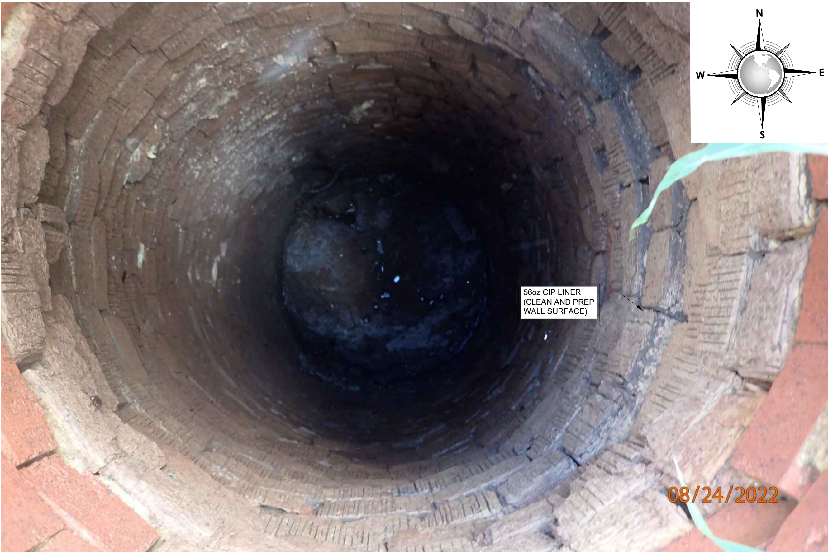
2 SANITARY SEWER MANHOLE 67 INTERIOR REHABILITATION PLAN (PHOTO) C67 C67 SCALE : N.T.S.
