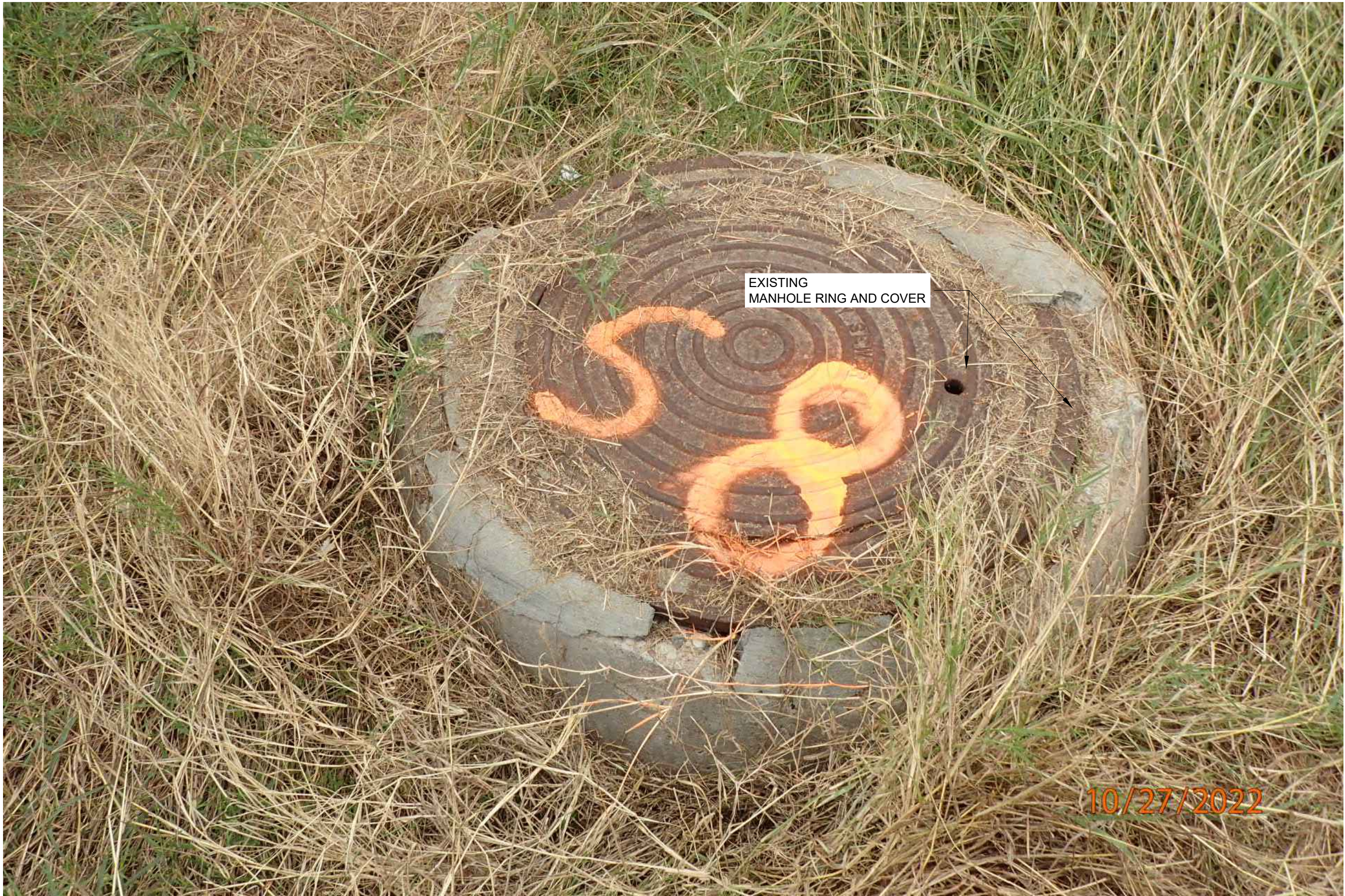
1 C58C58 SANITARY SEWER MANHOLE 58 EXTERIOR REHABILITATION PLAN (PHOTO) SCALE : N.T.S.
