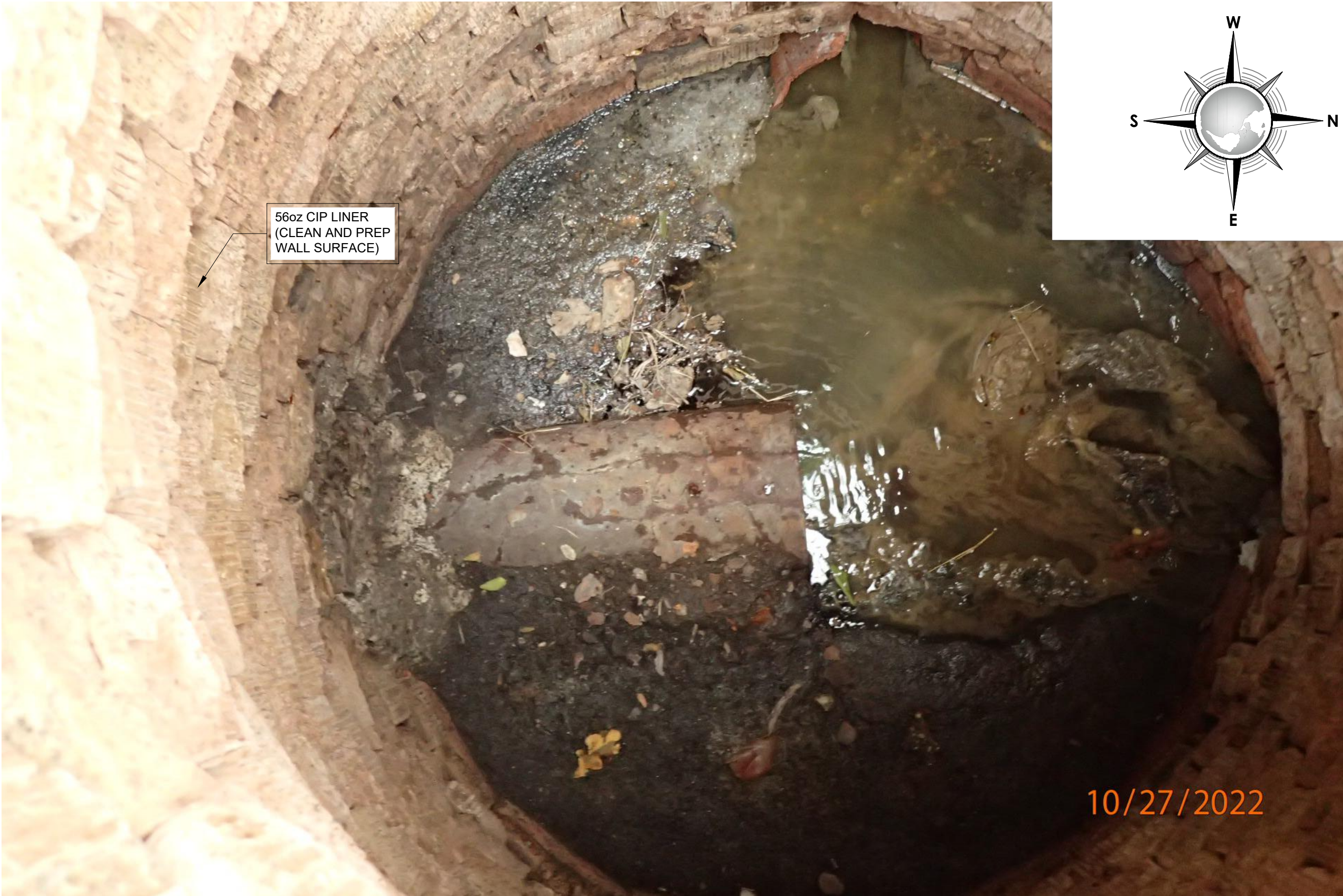
2 SANITARY SEWER MANHOLE 7 INTERIOR REHABILITATION PLAN (PHOTO) C10 C10 SCALE : N.T.S.
