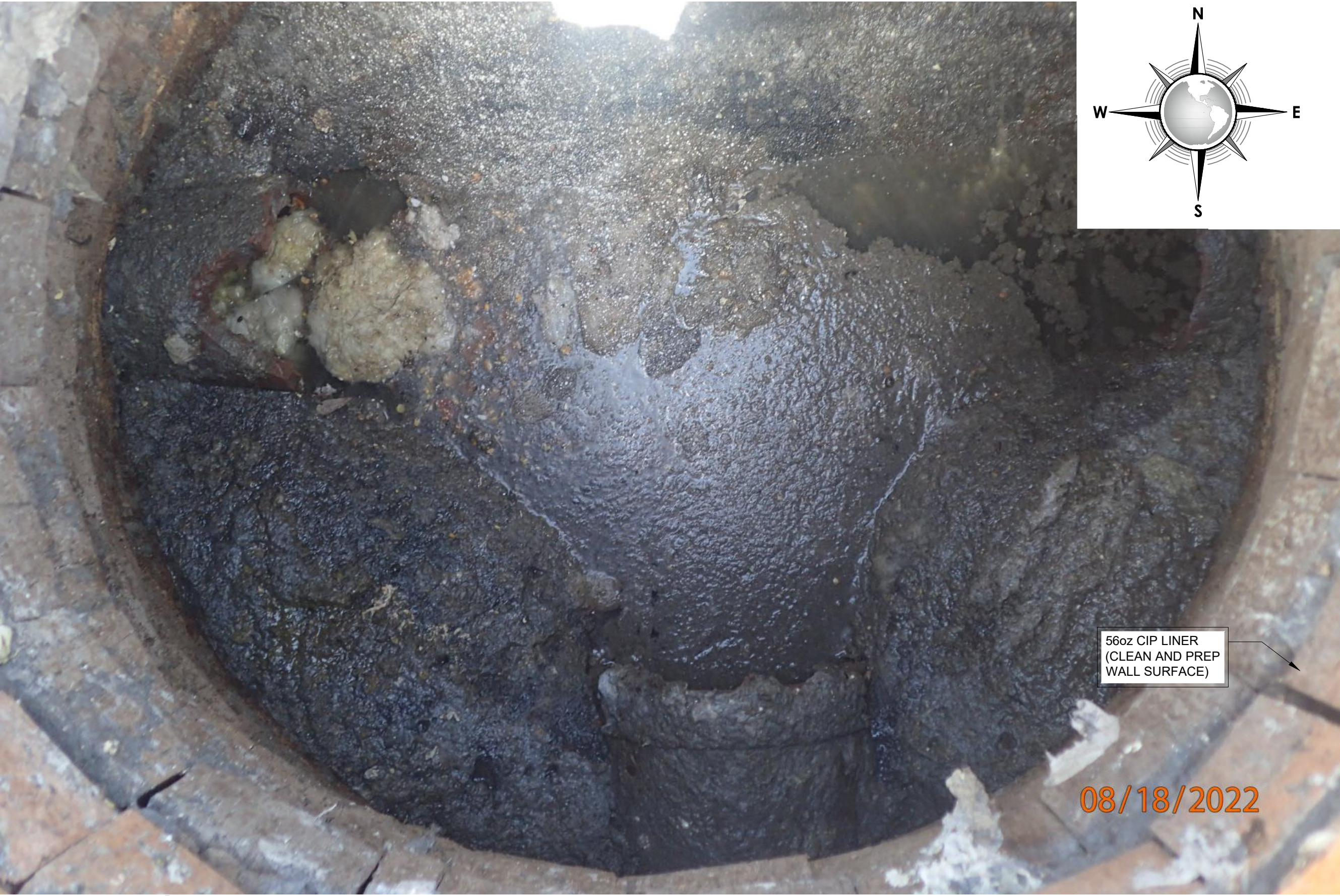
2 C41C41 SANITARY SEWER MANHOLE 41 INTERIOR REHABILITATION PLAN (PHOTO) SCALE : N.T.S.
