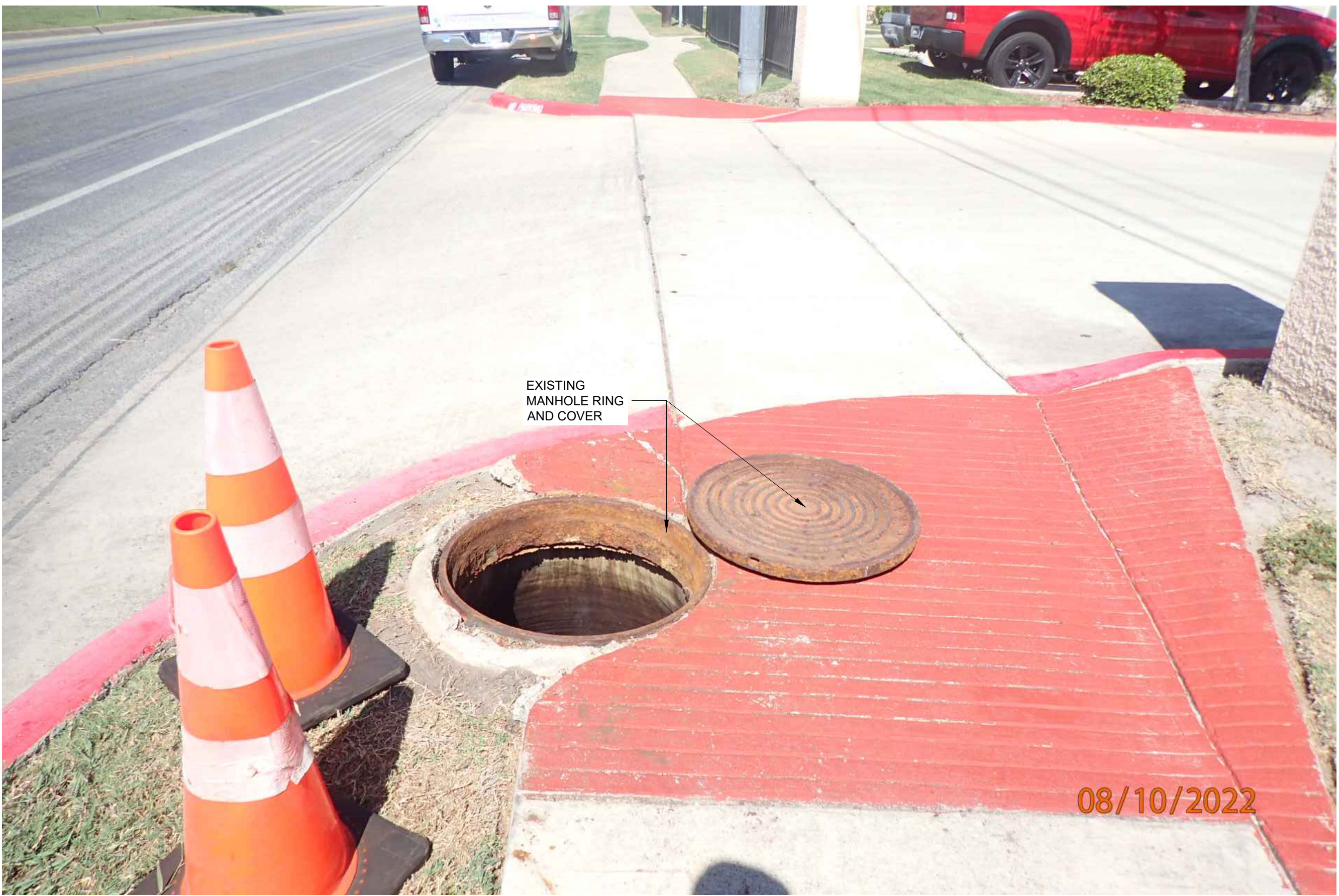
1 C13 C13 SANITARY SEWER MANHOLE 10 EXISTING EXTERIOR REHABILITATION PLAN (PHOTO) SCALE : N.T.S.
