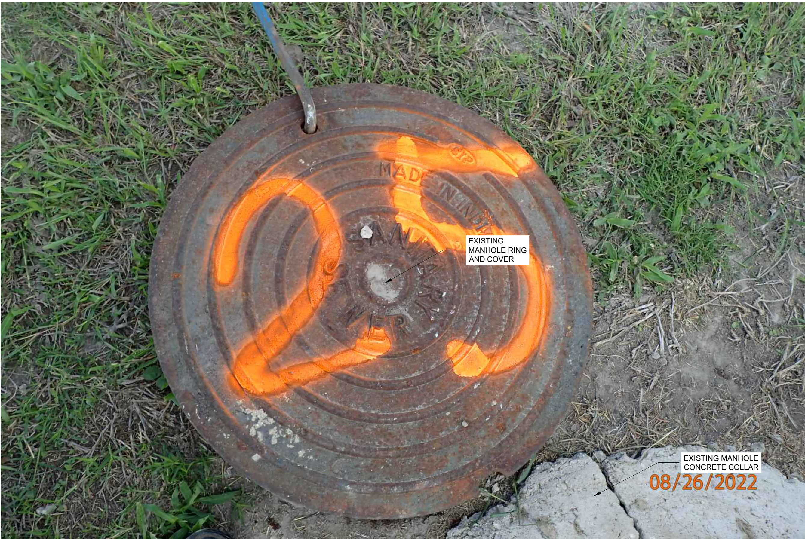
1 SANITARY SEWER MANHOLE 25 EXTERIOR REHABILITATION PLAN (PHOTO) SCALE : N.T.S.
