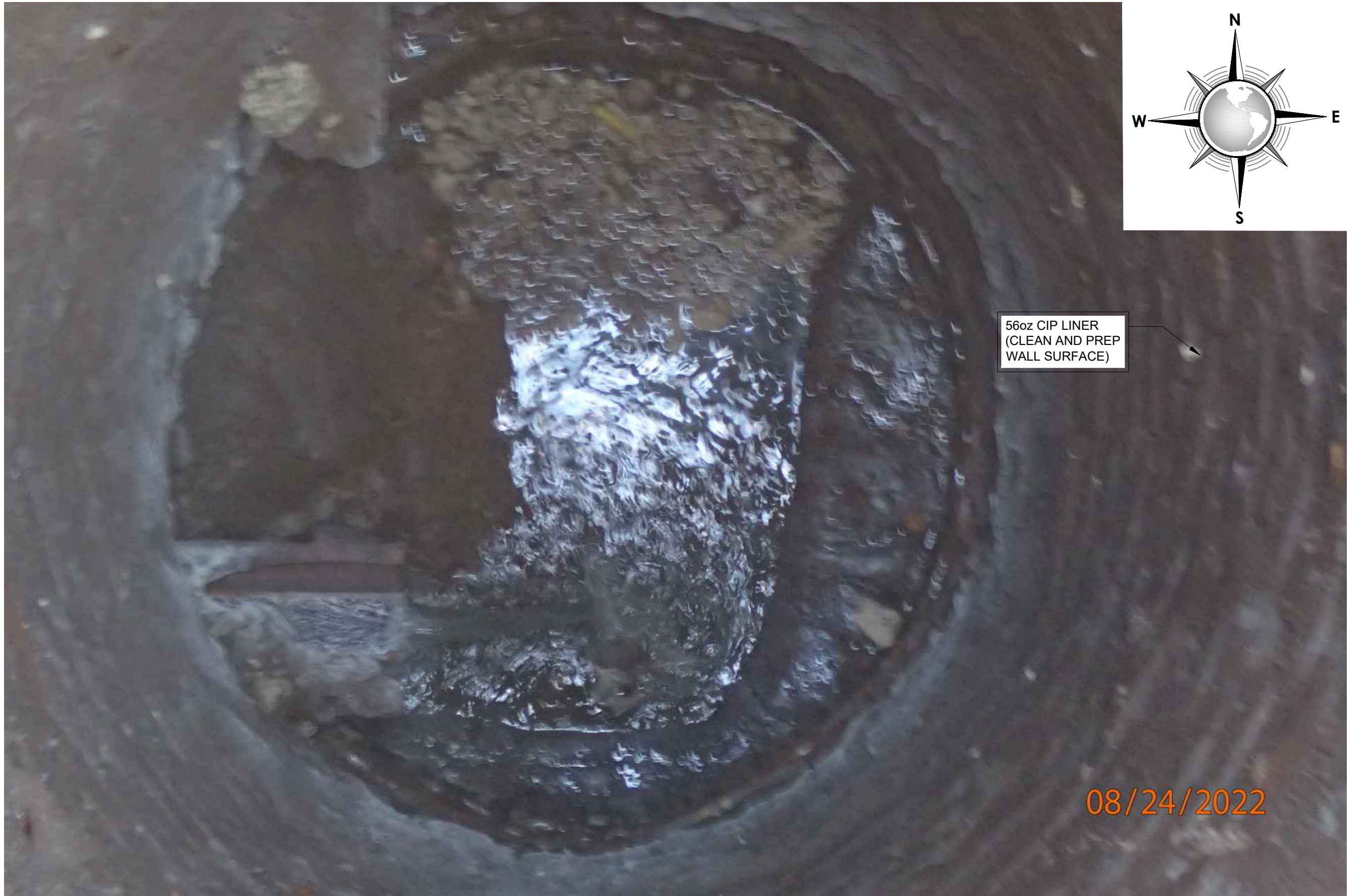
2 C65C65 SANITARY SEWER MANHOLE 65 INTERIOR REHABILITATION PLAN (PHOTO) SCALE : N.T.S.
