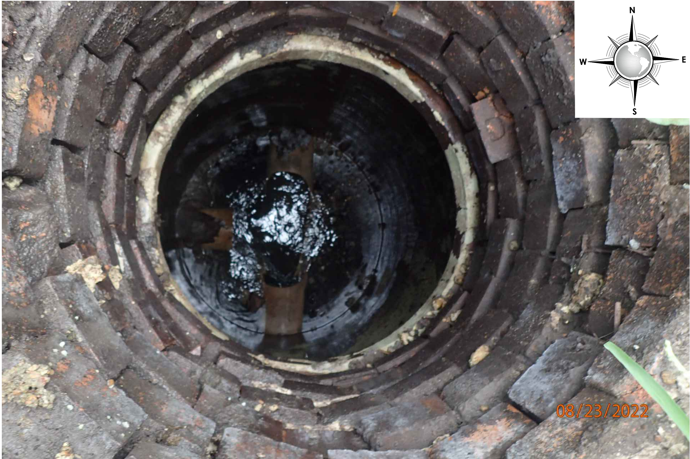
2 C59C59 SANITARY SEWER MANHOLE 59 INTERIOR REHABILITATION PLAN (PHOTO) SCALE : N.T.S.
