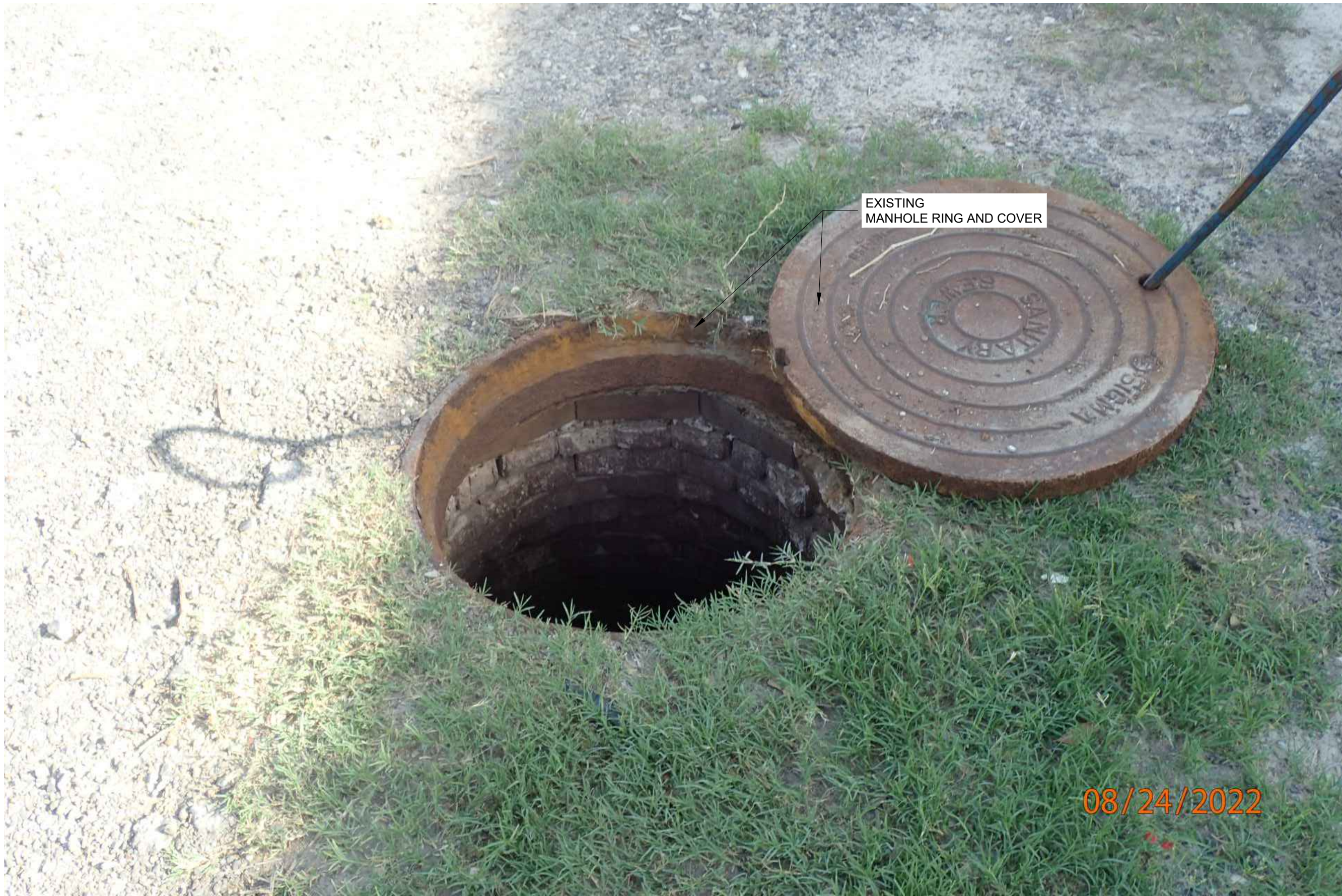
1 C65C65 SANITARY SEWER MANHOLE 65 EXTERIOR REHABILITATION PLAN (PHOTO) SCALE : N.T.S.
