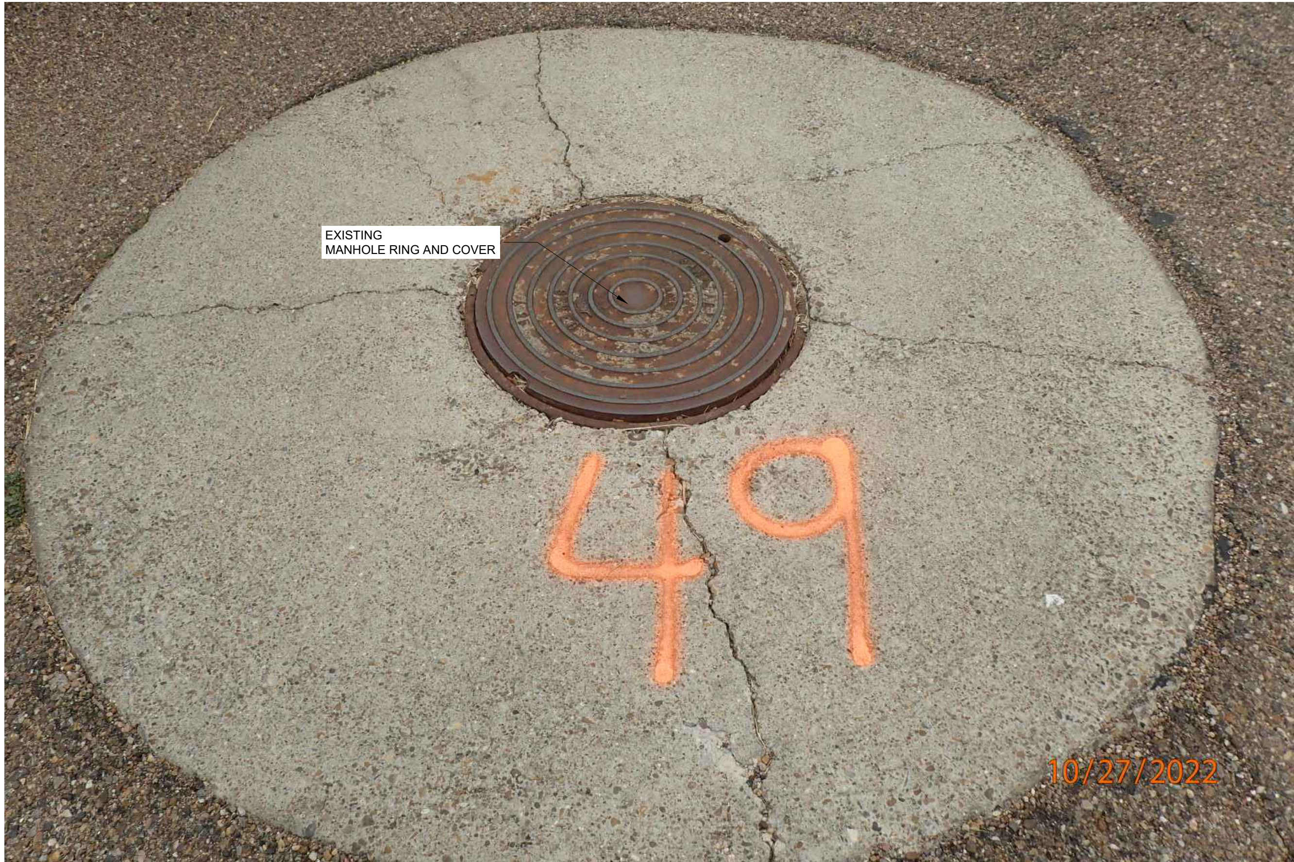
1 C49C49 SANITARY SEWER MANHOLE 49 EXTERIOR REHABILITATION PLAN (PHOTO) SCALE : N.T.S.
