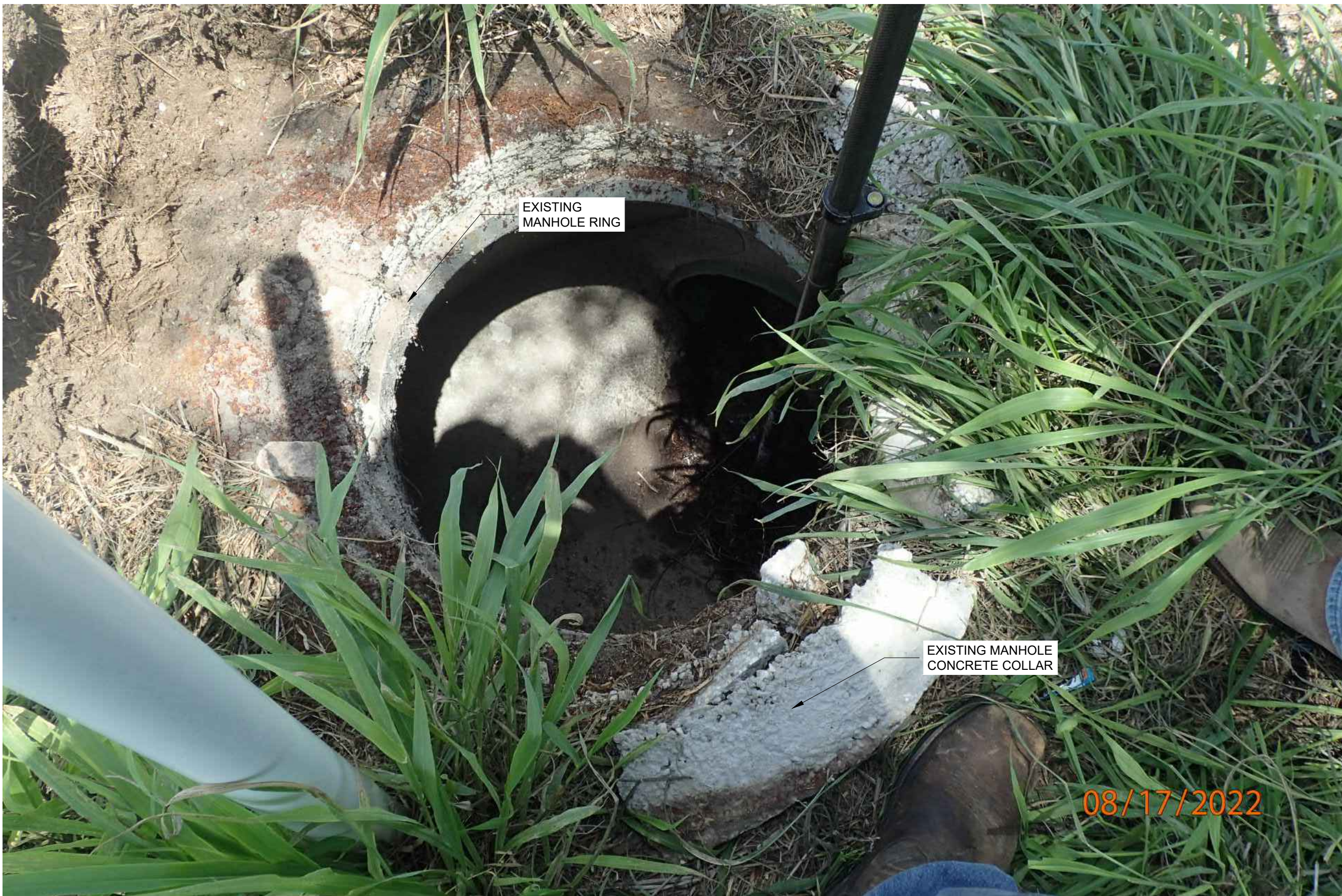
1 C38C38 SANITARY SEWER MANHOLE 38 EXTERIOR REHABILITATION PLAN (PHOTO) SCALE : N.T.S.
