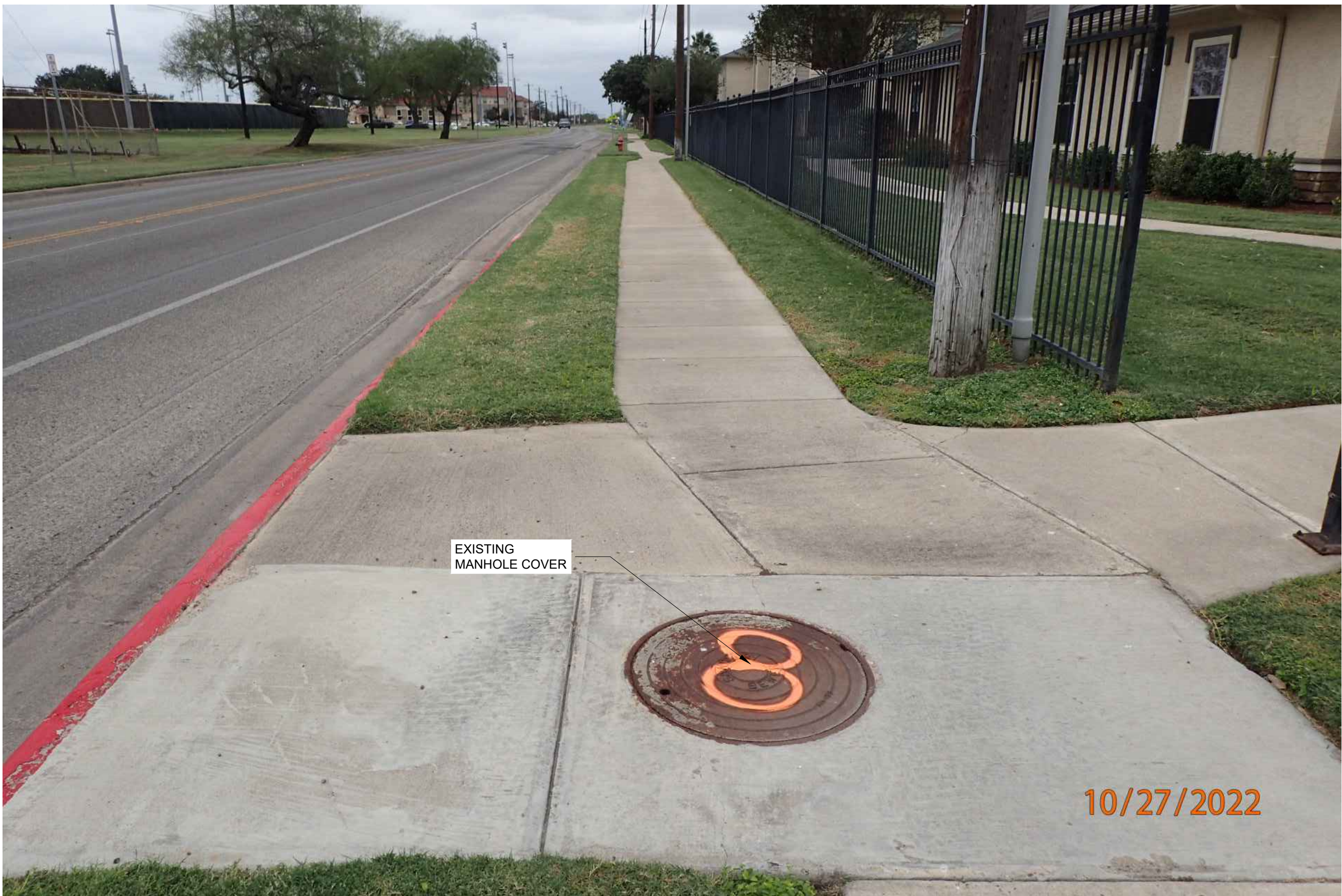
1 SANITARY SEWER MANHOLE 8 EXISTING EXTERIOR REHABILITATION PLAN (PHOTO) C11 C11 SCALE : N.T.S.
