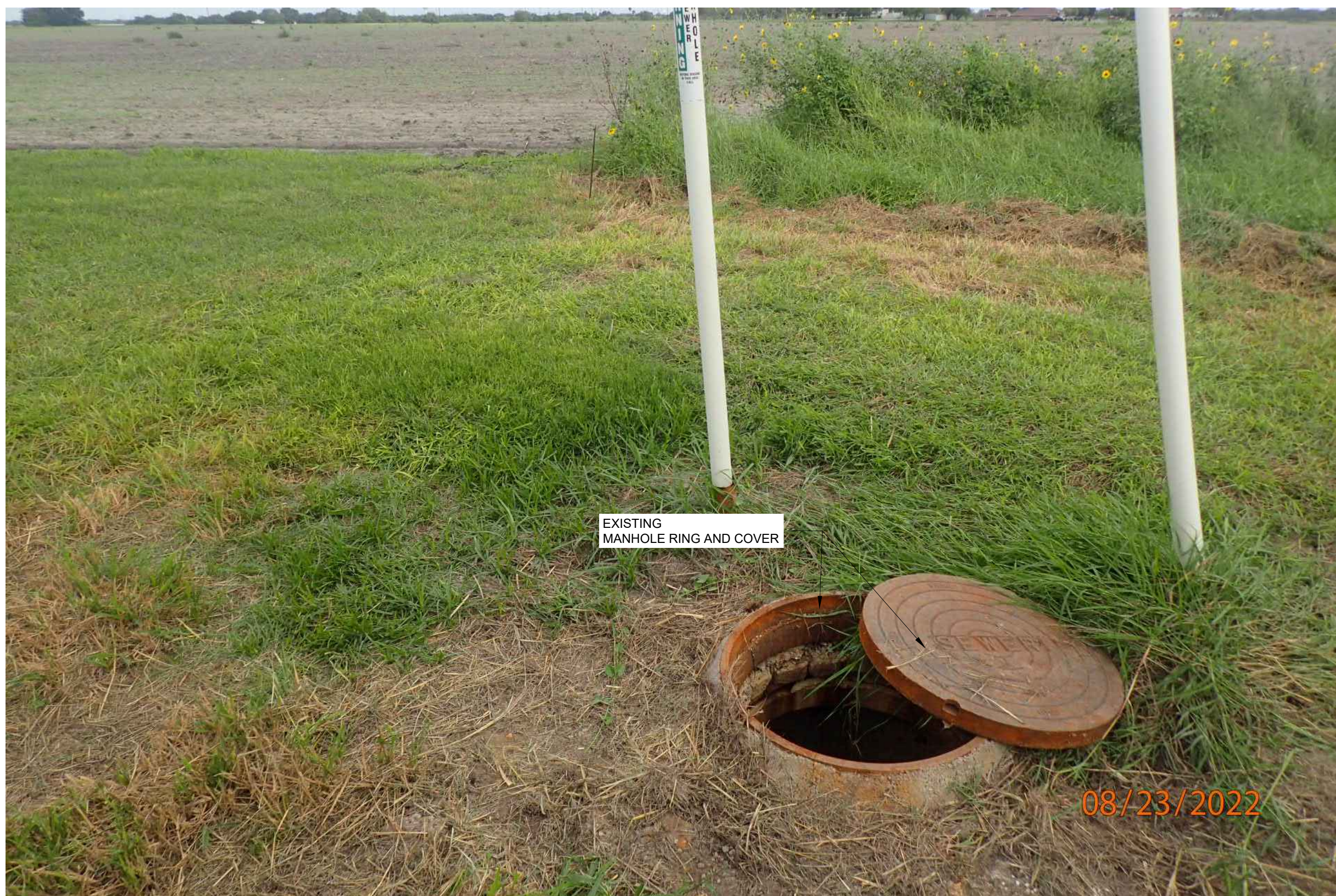
1 SANITARY SEWER MANHOLE 60 EXTERIOR REHABILITATION PLAN (PHOTO) C60 C60 SCALE: N.T.S.
