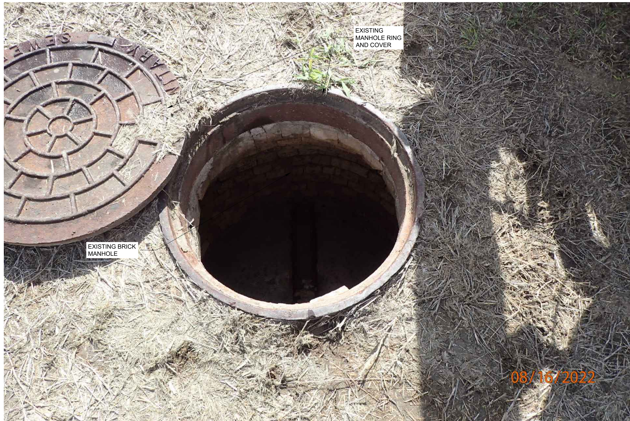
1 SANITARY SEWER MANHOLE 29 EXISTING EXTERIOR REHABILITATION PLAN (PHOTO) C29 C29 SCALE: N.T.S.
