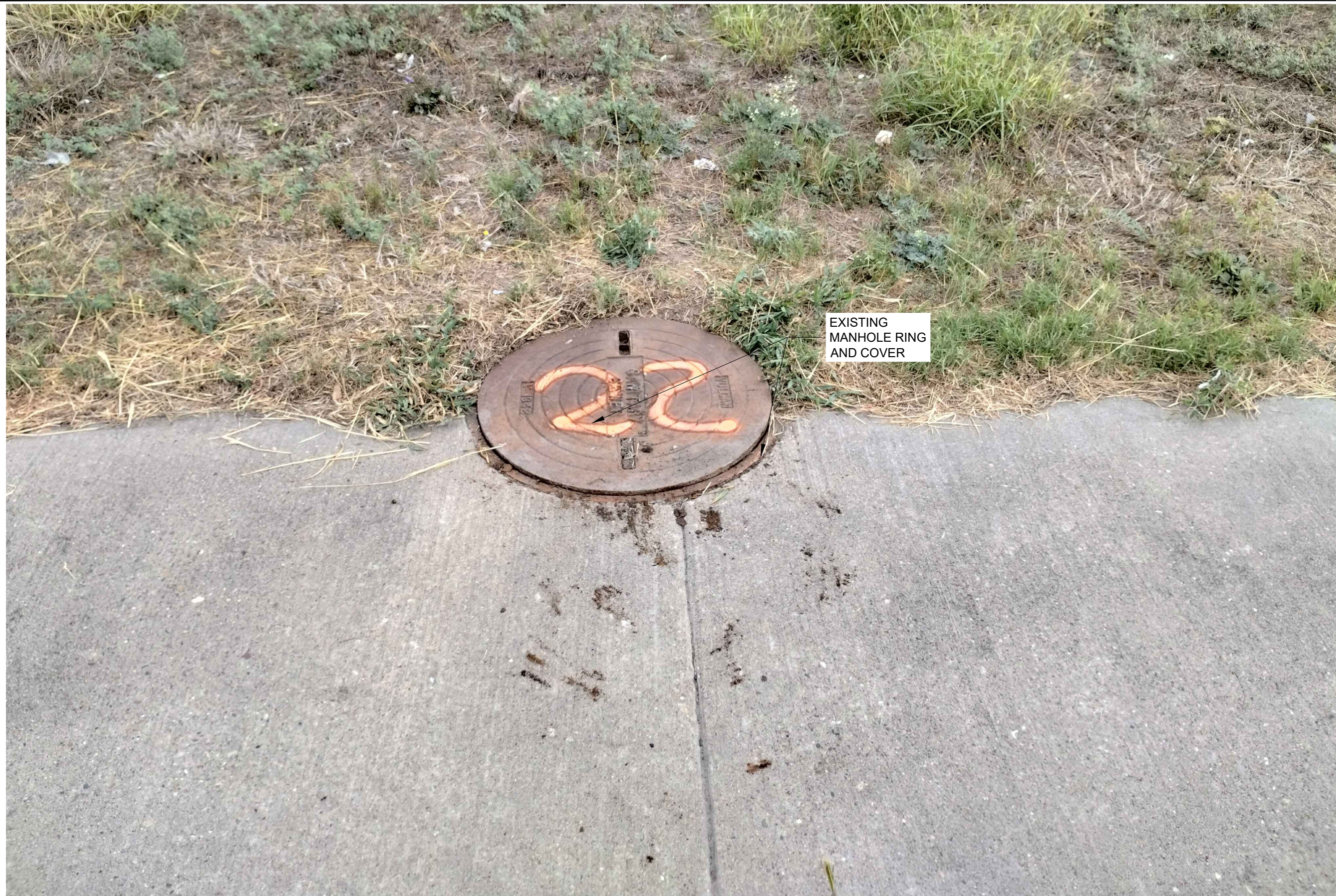
1 SANITARY SEWER MANHOLE 22 EXTERIOR REHABILITATION PLAN (PHOTO) C24 C24 SCALE: N.T.S.
