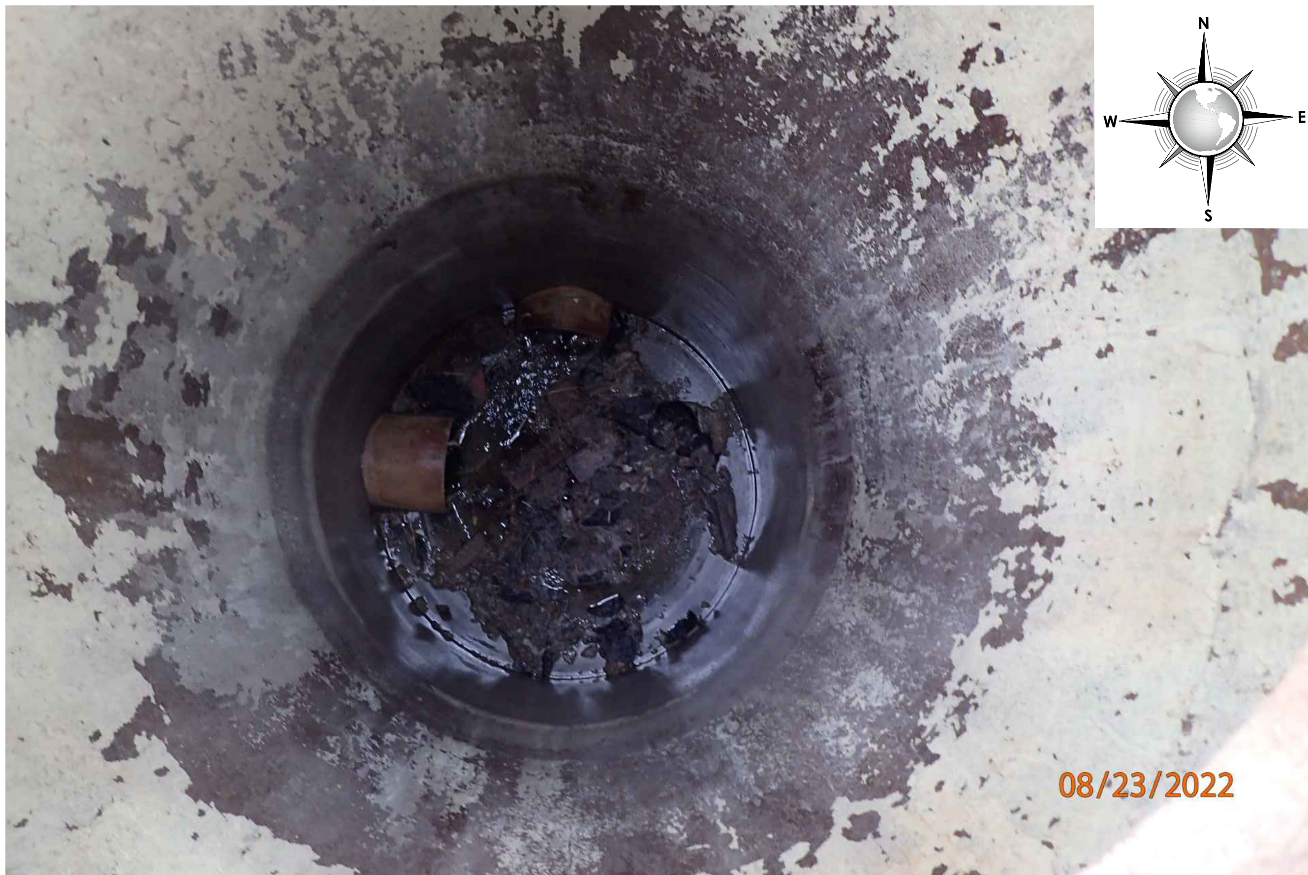
2 SANITARY SEWER MANHOLE 60 INTERIOR REHABILITATION PLAN (PHOTO) C60 C60 SCALE: N.T.S.
