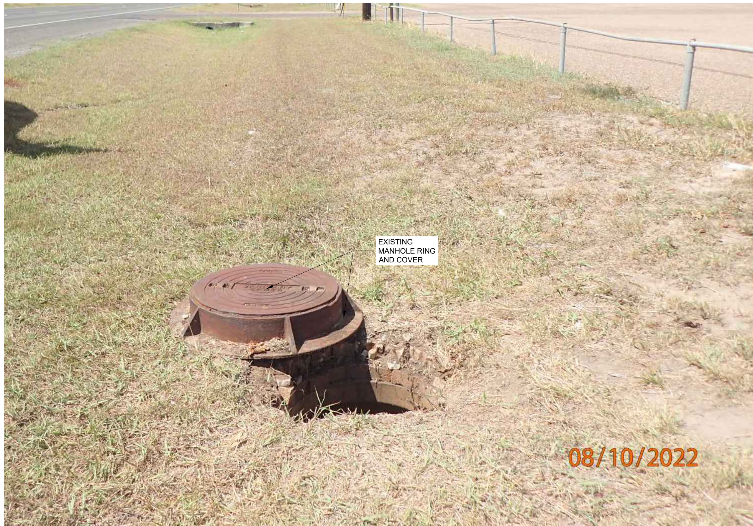
1 SANITARY SEWER MANHOLE 16 EXTERIOR REHABILITATION PLAN (PHOTO) C19 C19 SCALE: N.T.S.
