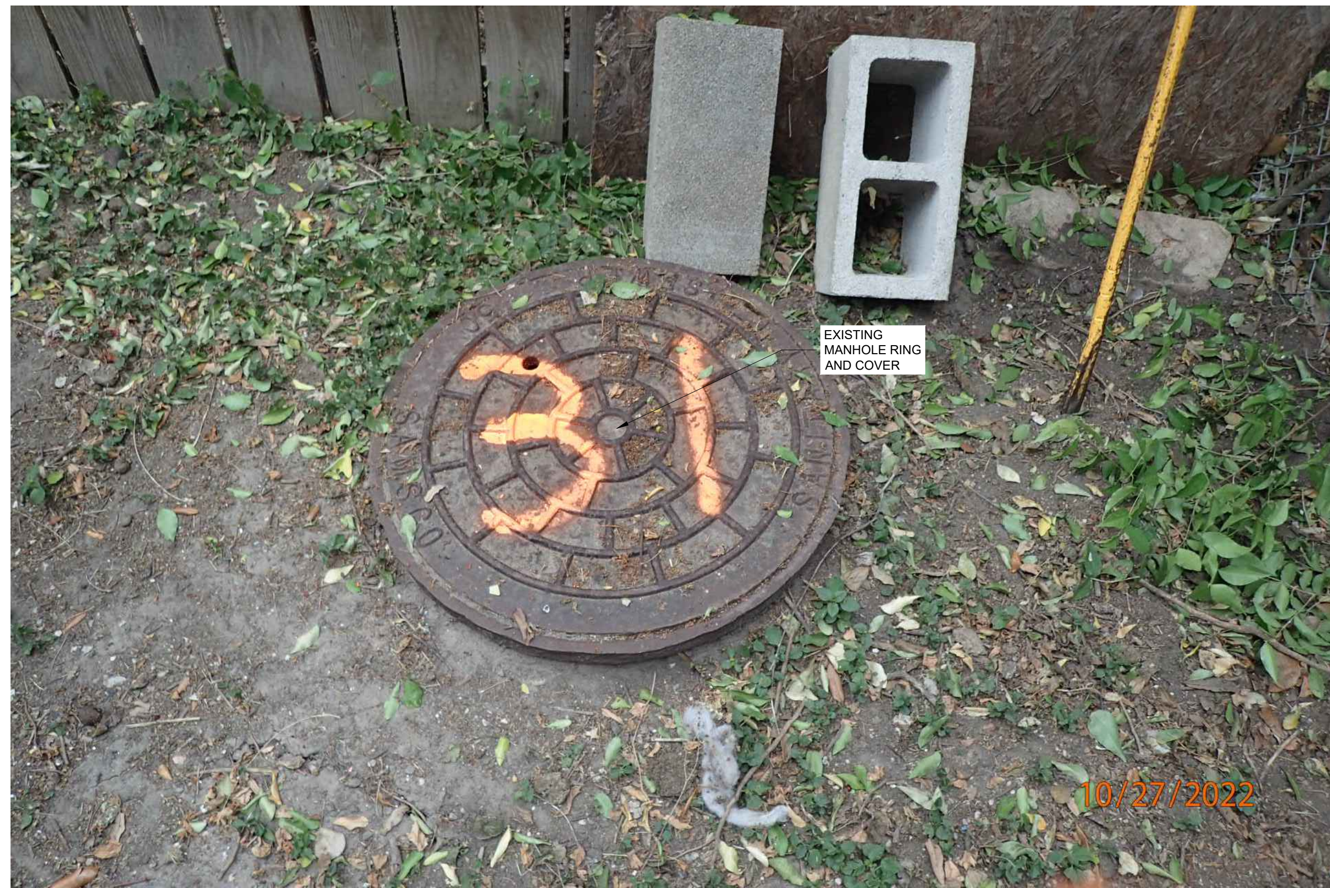
1 SANITARY SEWER MANHOLE 31 EXISTING EXTERIOR REHABILITATION PLAN (PHOTO) C31 C31 SCALE: N.T.S.
