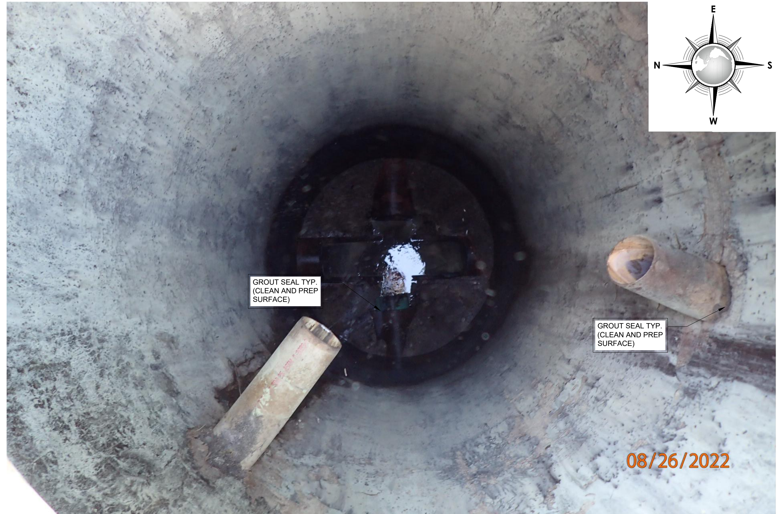
2 SANITARY SEWER MANHOLE 39 INTERIOR REHABILITATION PLAN (PHOTO) C39 C39 SCALE: N.T.S.
