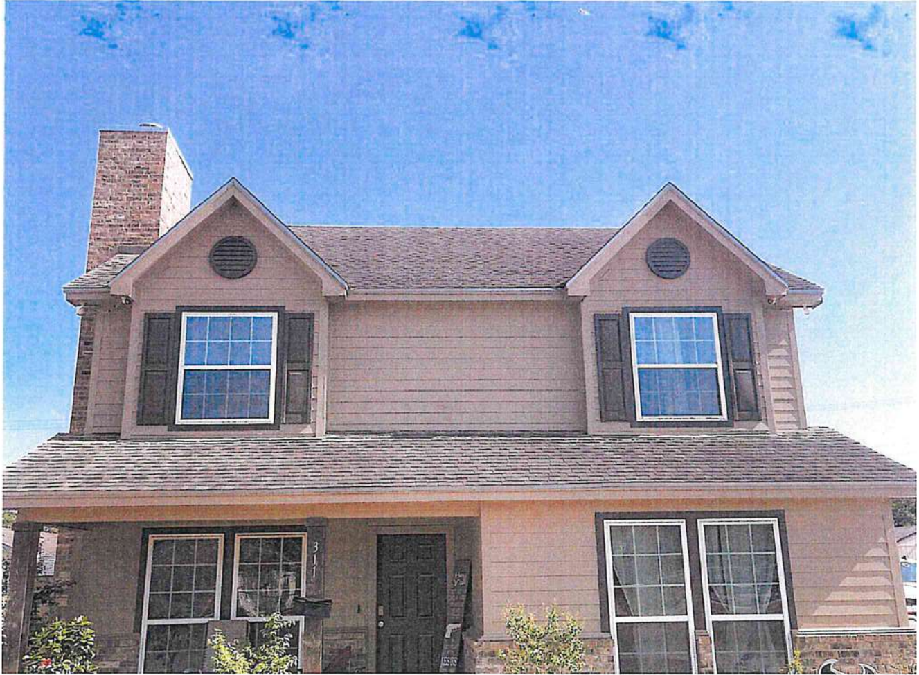
Insulation LLC Loc: 27.5227, -97.8657
